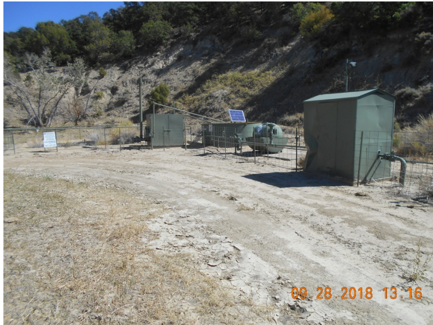
Meter housing, Separator and blowdown tank.
