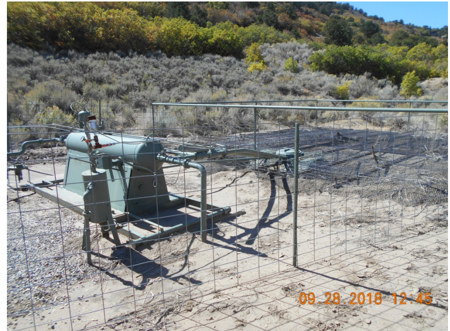
05-077-08311 Separator and blowdown tank
