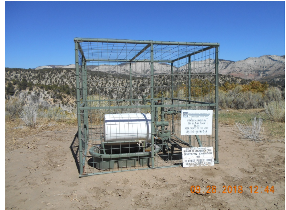
05-077-08311 Wellhead with fence and sign
