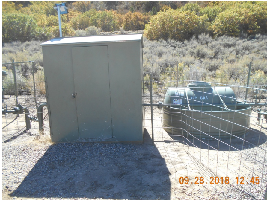
05-077-08311 Meter housing and chemical tank
