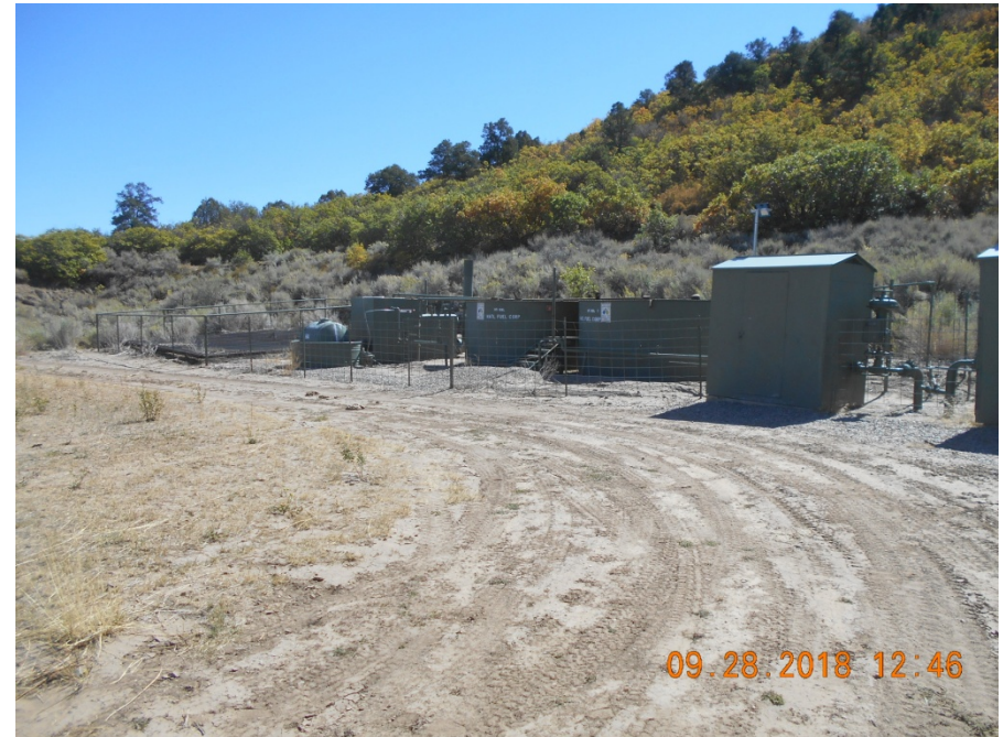
05-077-08318 Separator, Tank battery, meter housing and blowdown tank
