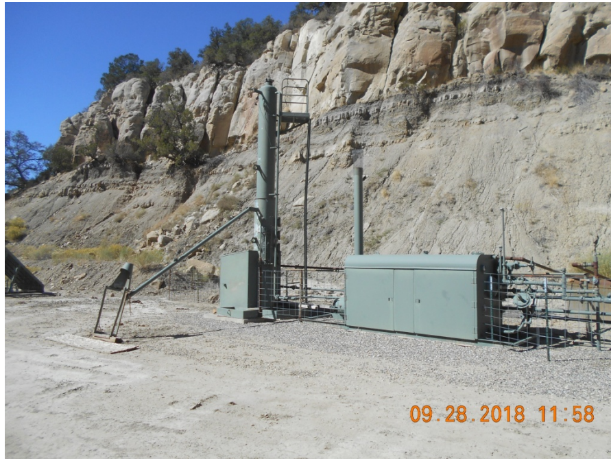
Separator and Dehydrator
