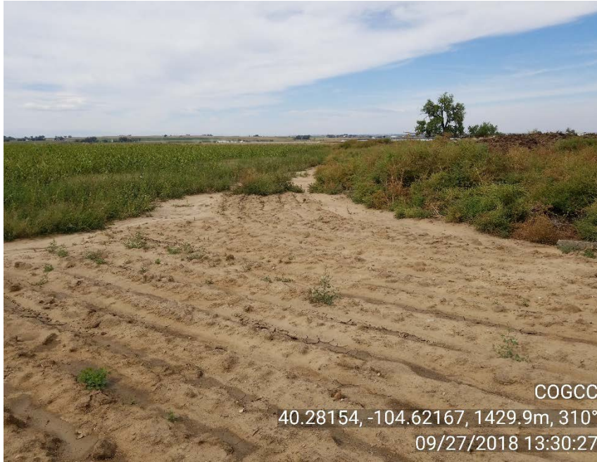
Photo 3 – Sediment transported off-site in NE corner
