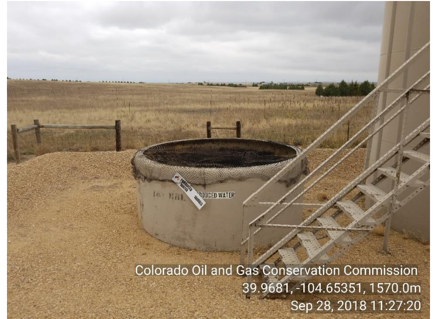
Photo 4 Bird netting repaired
