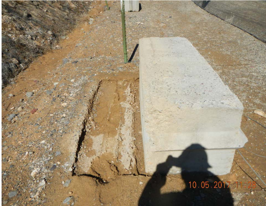
Deadman anchor dragged towards pit. Looking NNW
