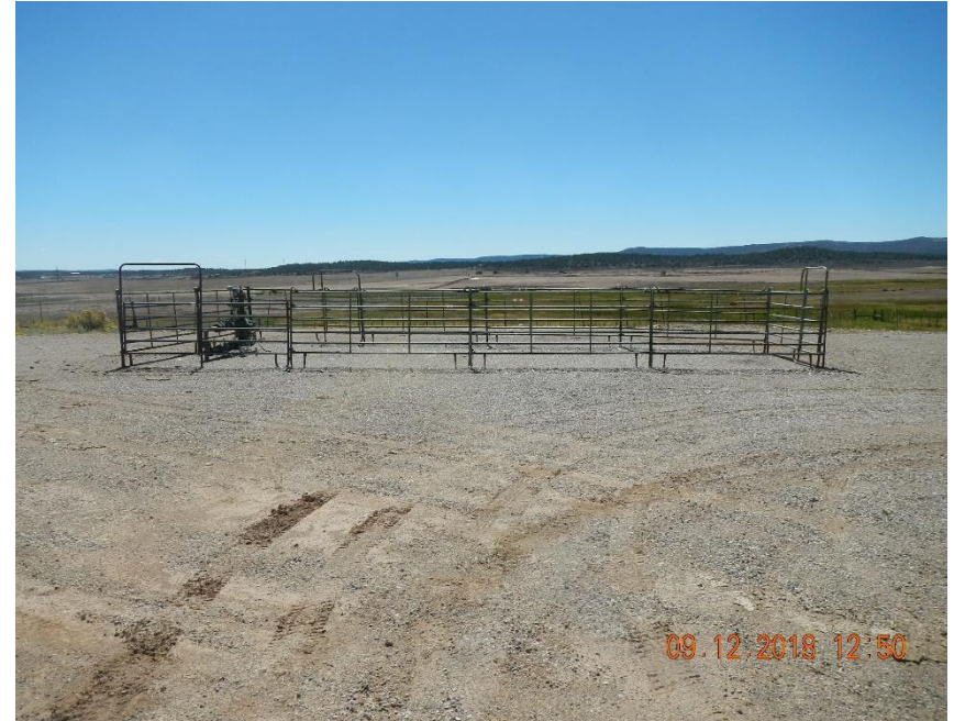
Stock panel enclosure around well head.
