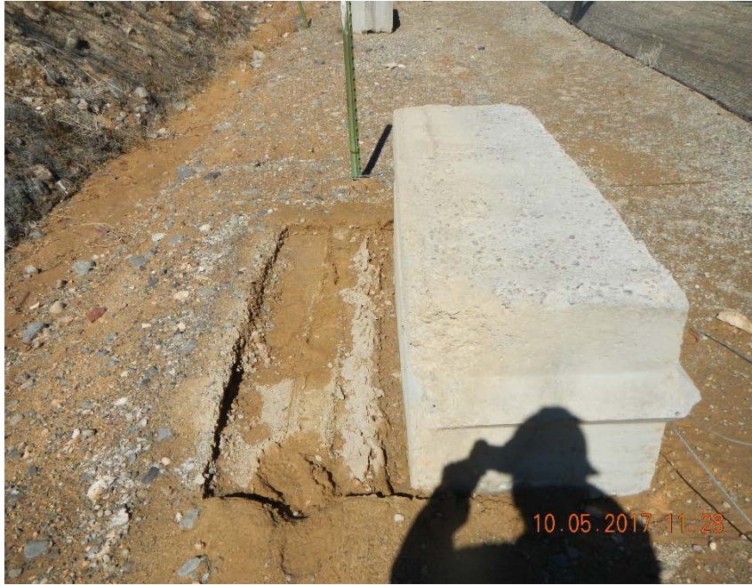
Deadman anchor dragged towards pit. Looking NNW
