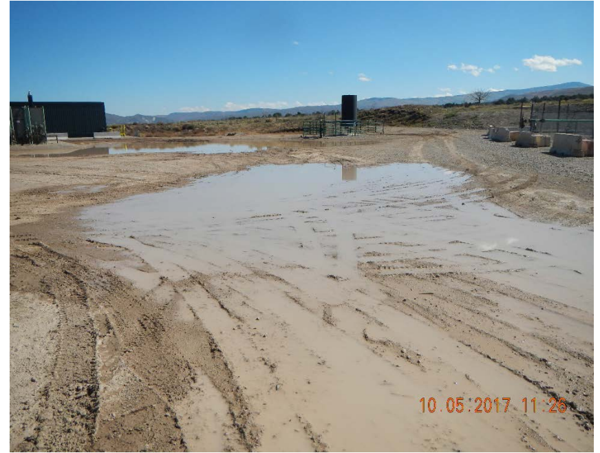
Snowmelt standing water on pad, looking east
