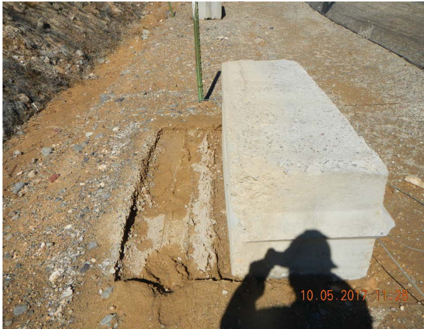
Deadman anchor dragged towards pit. Looking NNW
