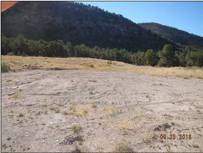
Photo 1: Well has been plugged and cut off.
