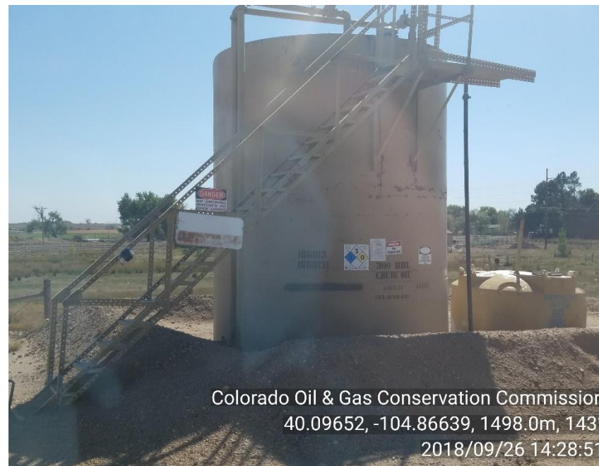
PHOTO 2: TANK BATTERY
