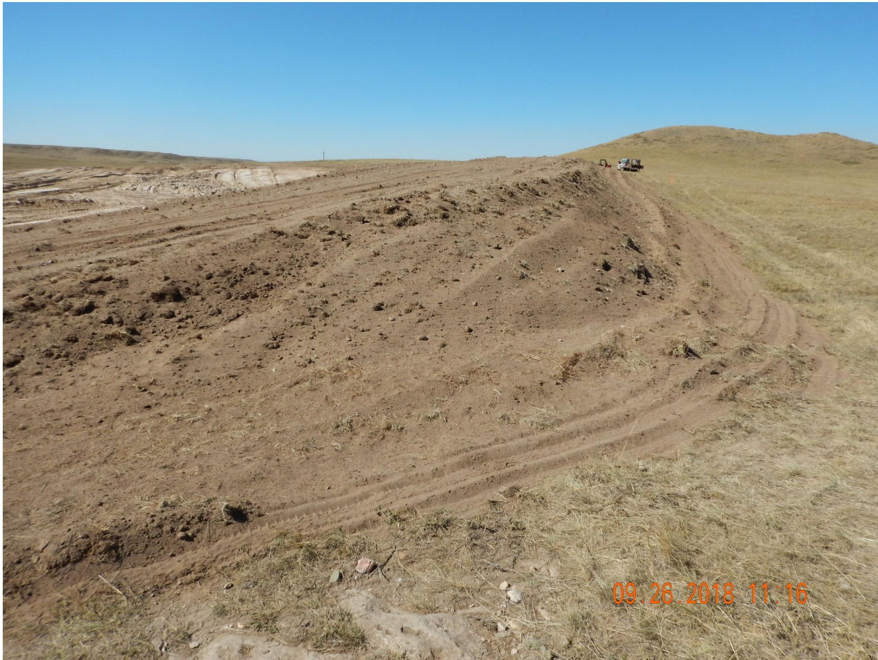
Photo 2. Photo taken from the northeastern perimeter of the location, facing West. Operator has salvaged and stored the topsoil along the northern perimeter. Operator plans to seed and mulch topsoil.
