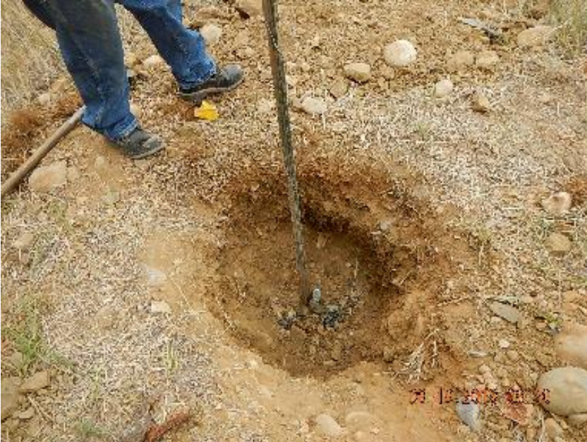
Photo 5: T post and tracer wire.
