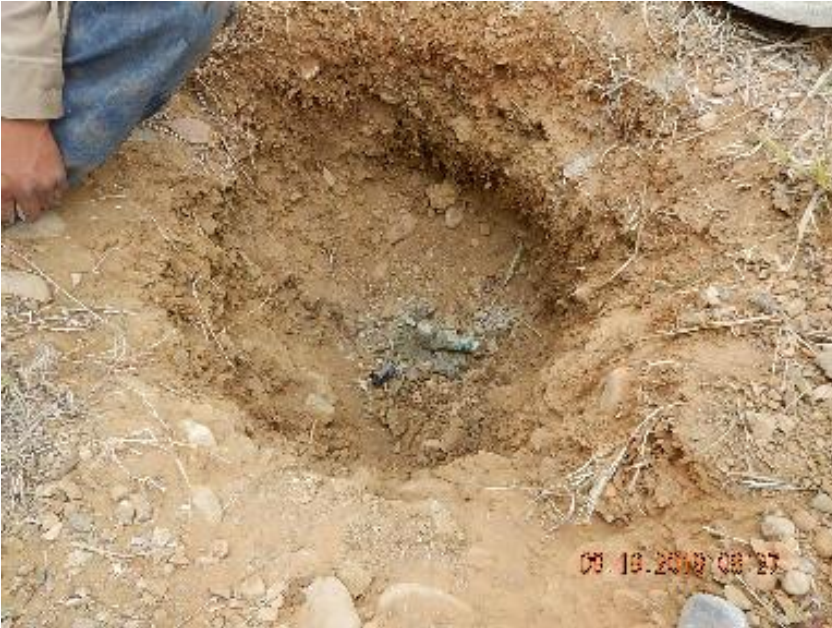
Photo 3: Line filled with concrete and plugged.
