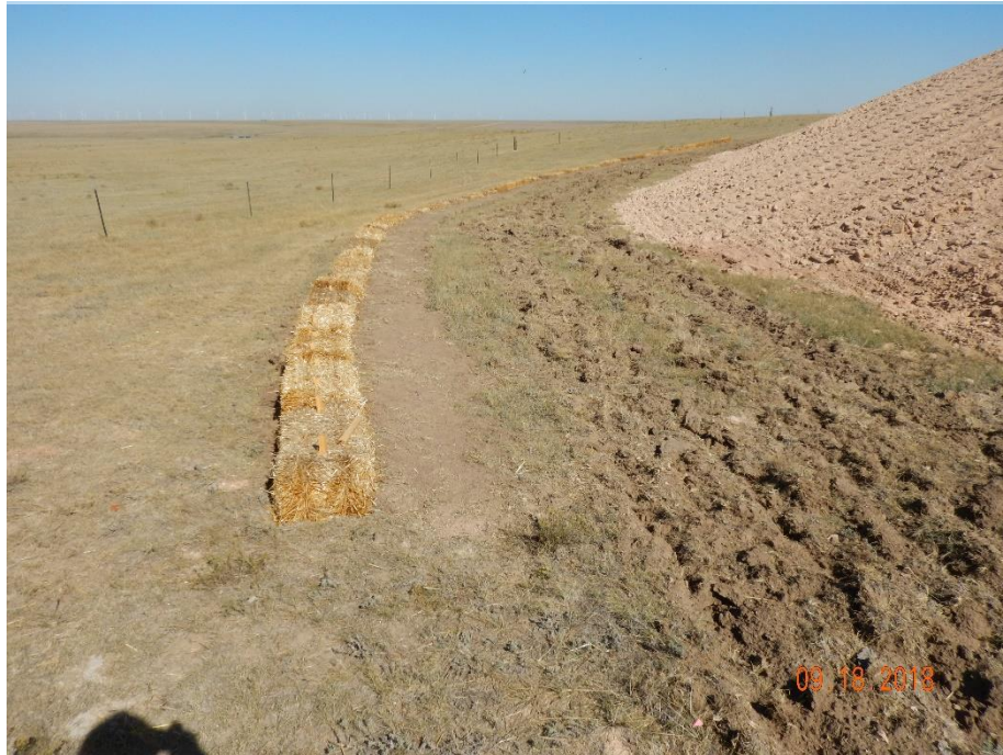
Photo 3: Photo taken from the southwest corner of the location, facing north. Photo shows bales have been installed as a stormwater/erosion control BMP. BMPs appears to have been installed in accordance with good engineering practices. Photo also shows surface roughening along perimeter appears to have been updated/maintained.
