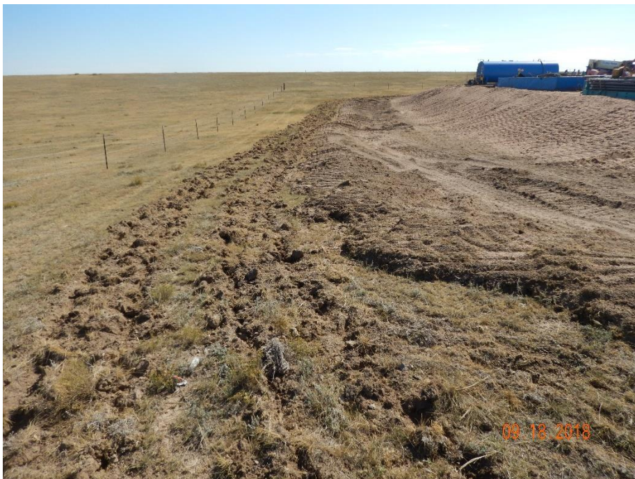
Photo 5: Photo taken from the northwest corner of the location, facing east. Photo shows operator has implemented berms along the perimeter of the pad, and another on the perimeter of the location. Surface roughening has been used in conjunction.
