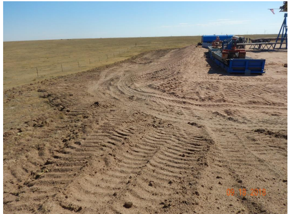
Photo 4: Photo taken from the northwest corner of the pad, facing east. Photo shows operator has implemented berms along the perimeter of the pad, and another on the perimeter of the location. Surface roughening has been used in conjunction.
