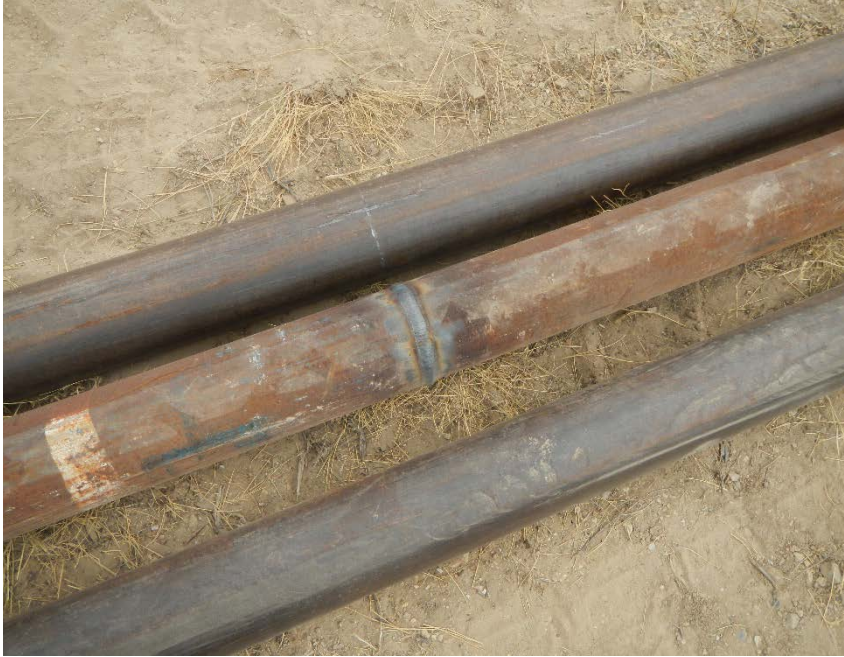
New welded pipeline segment
