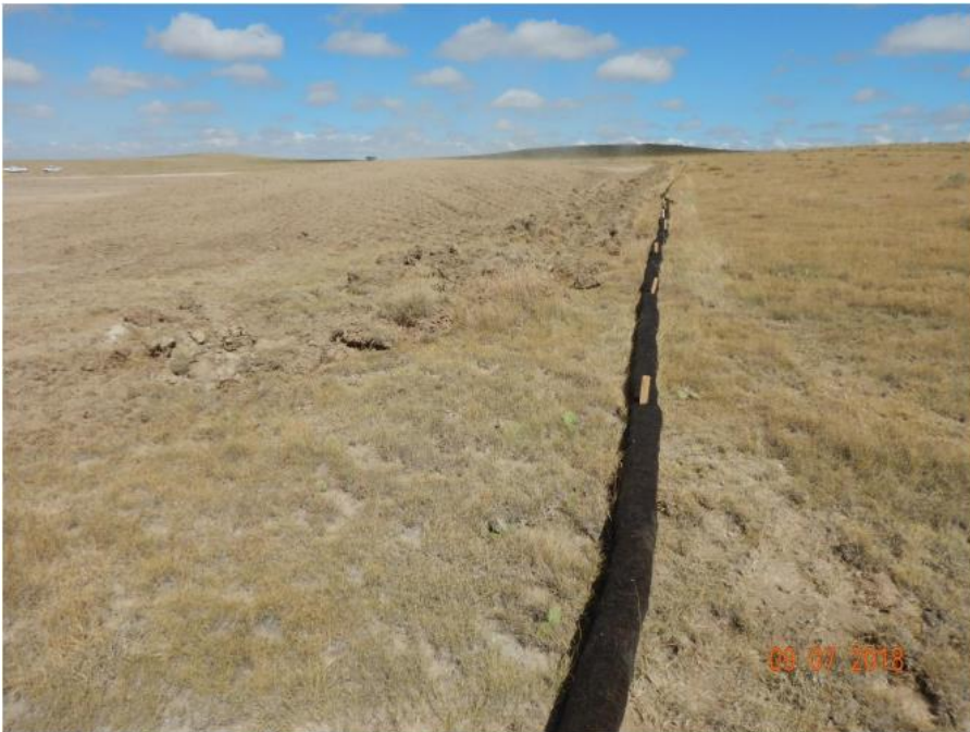
Photo 12: Photo taken from the northeast corner of the location, facing north. Photo shows topsoil stockpile for the location. Contractors performing soil salvage and construction indicate that "~4-6 inches of topsoil" was salvaged and stored on the southeast end of the location. It does not appear as though sufficient topsoil salvage has been conducted on the location.
