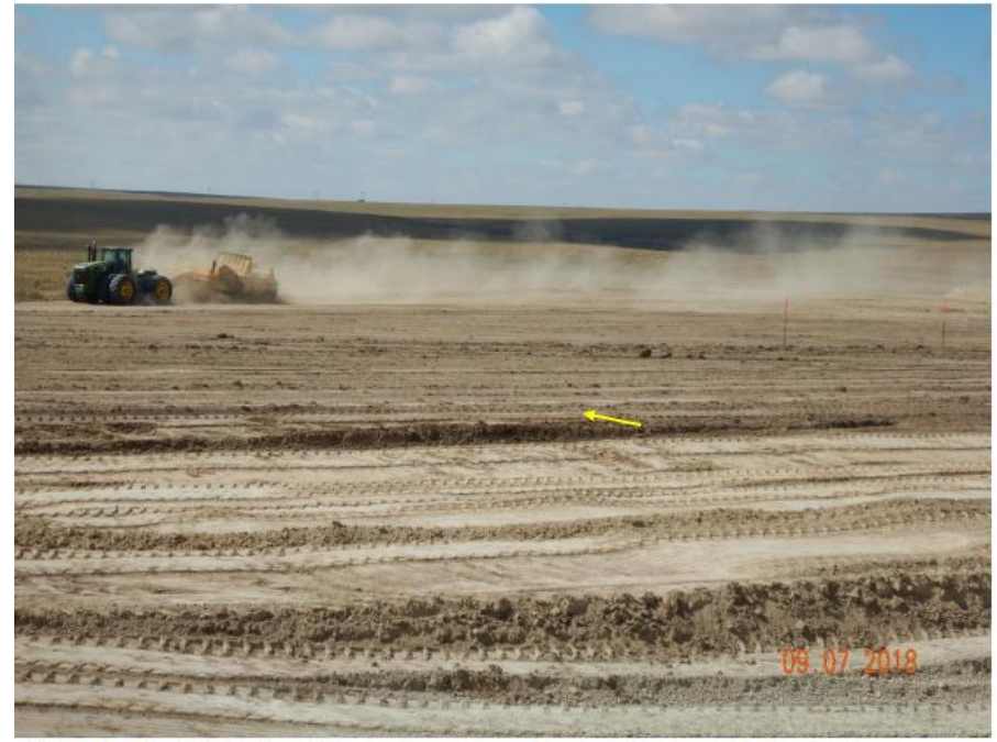
Photo 15: Photo taken from the northern area of the pad, facing south. Photo shows unsalvaged topsoil appears to remain on the pad.. It was observed that the scraper collected soils (photo 14) from areas of the pad for fill material on the southern end of the location; it appears as though topsoil is being incorporated with subsoils as fill material. See comments under photo 13 and 14
