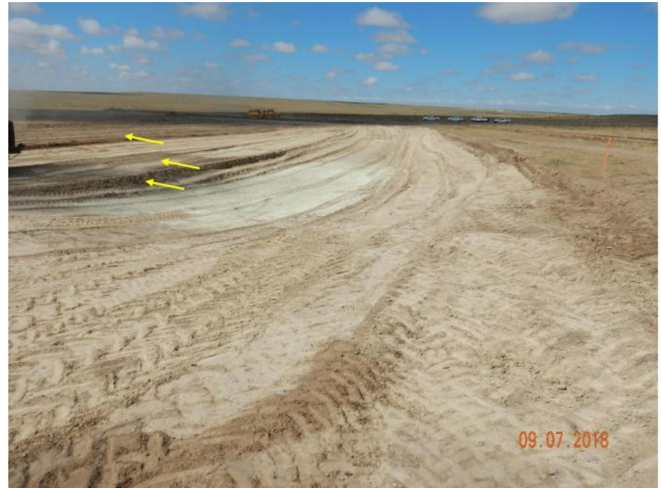
Photo 13: Photo taken from the southeast corner of the pad, facing west. Photo shows unsalvaged topsoil appears to remain on the pad.
