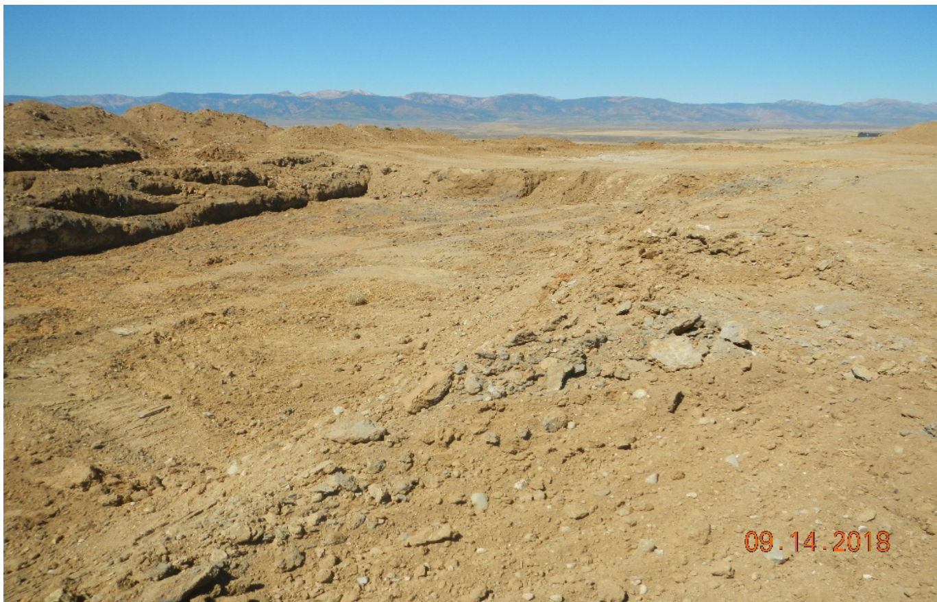
Photo#2: Remediation project #9817 in process at Location.
