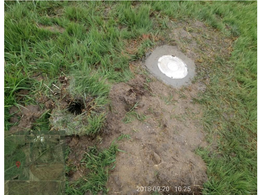
Photo 2 – Recently installed monitoring well.
