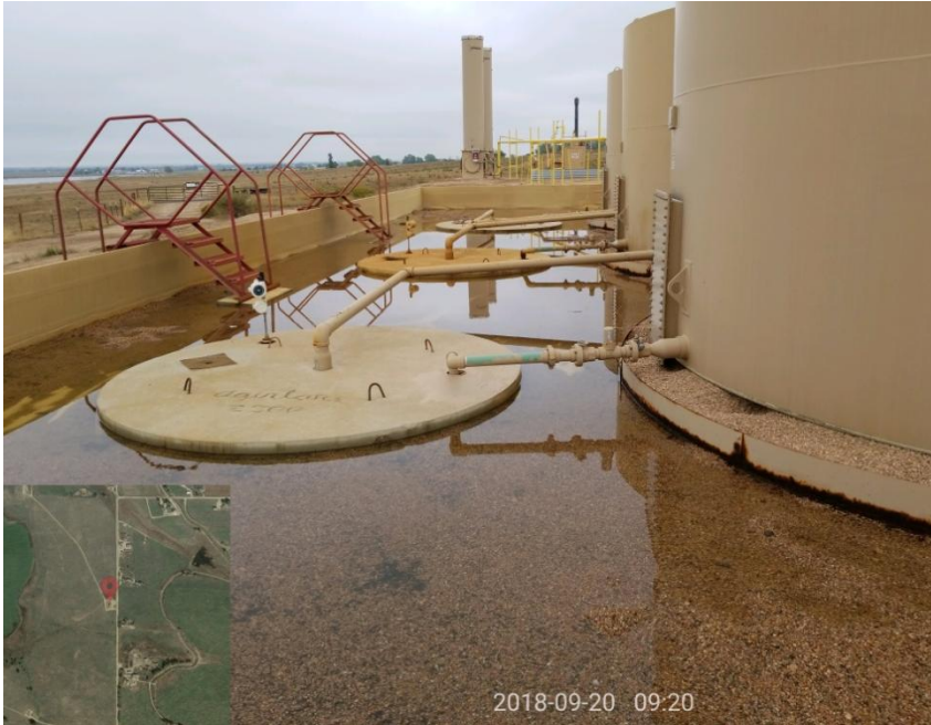
Photo 1 – Stormwater within lined tank berm from recent storms.
