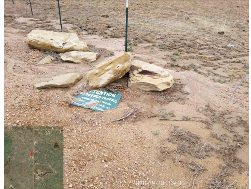
Photo 4 – Stormwater transported sediment and trash at south and west perimeters.
