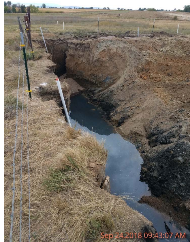
Photo 2 – Downgradient (south) edge of former Tank Battery and Wellhead footprint. Viewing groundwater amendments trench, looking west.
