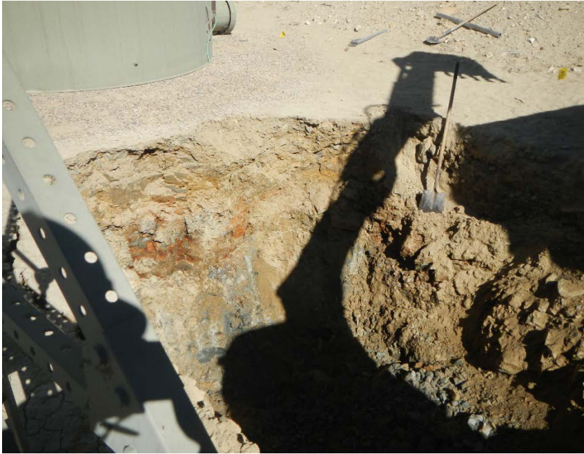
Pit looking NW
