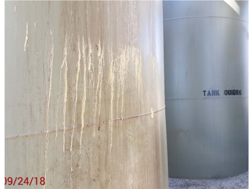
Location Photo #4, oily residue on sde of tanks.
