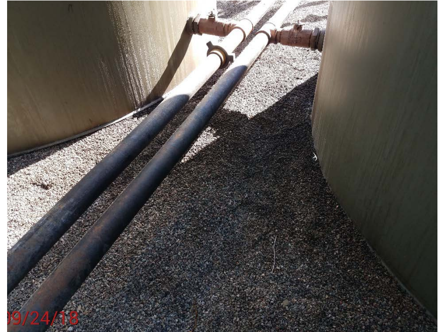
Location Photo #6, stained rock in battery containment.
