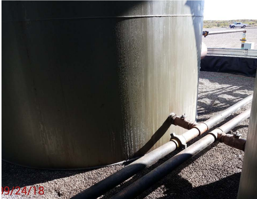
Location Photo #5, stained rock in battery containment.
