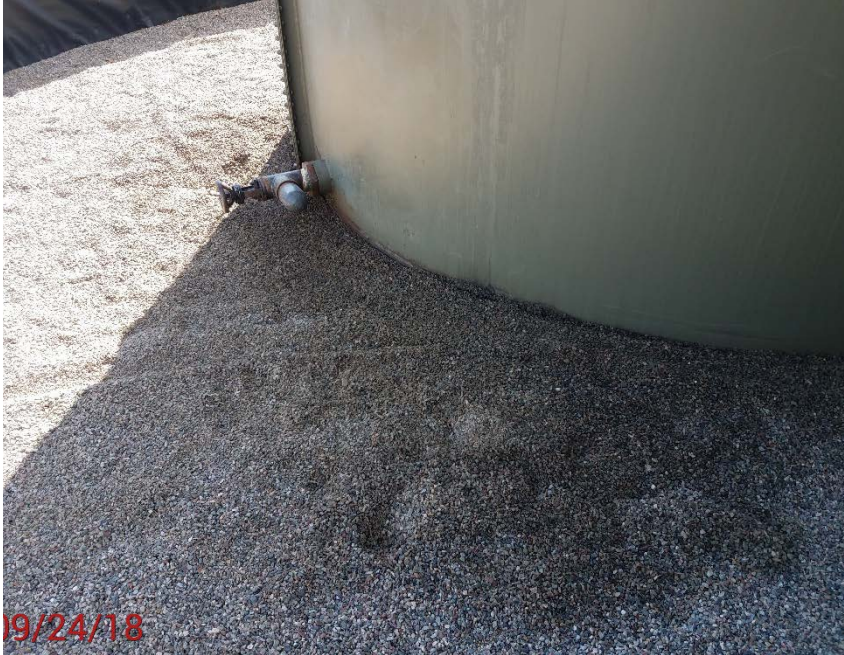
Location Photo #7, stained rock in battery containment.
