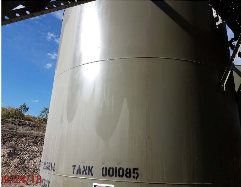
Location Photo #3, oily residue on side of tanks.
