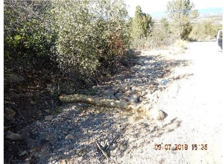
Photo 8: Access road check dam and rock installed at culvert.
