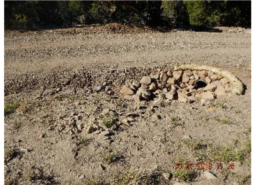
Photo 10: Culvert inflow along access road.
