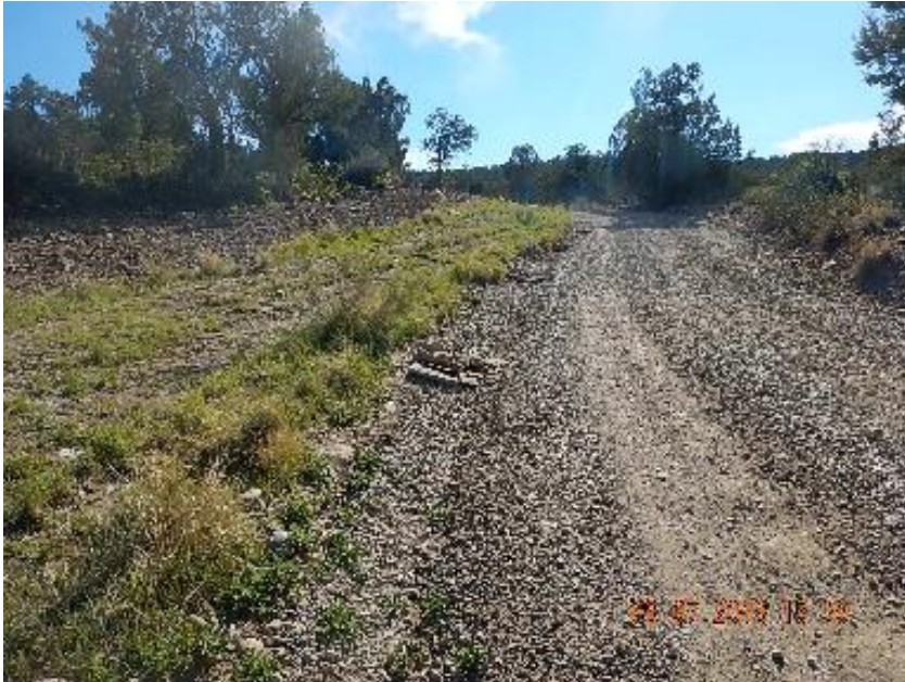
Photo 11: Check dams along access road.
