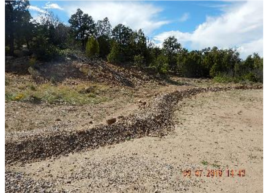
Photo 4: New berm added to the lower Jacques 1 location area.
