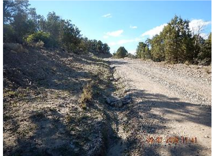
Photo 12: Check dams along access road.
