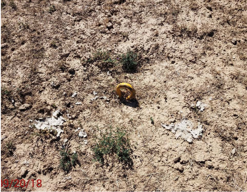
Location Photo #7, unmarked deadman anchor
