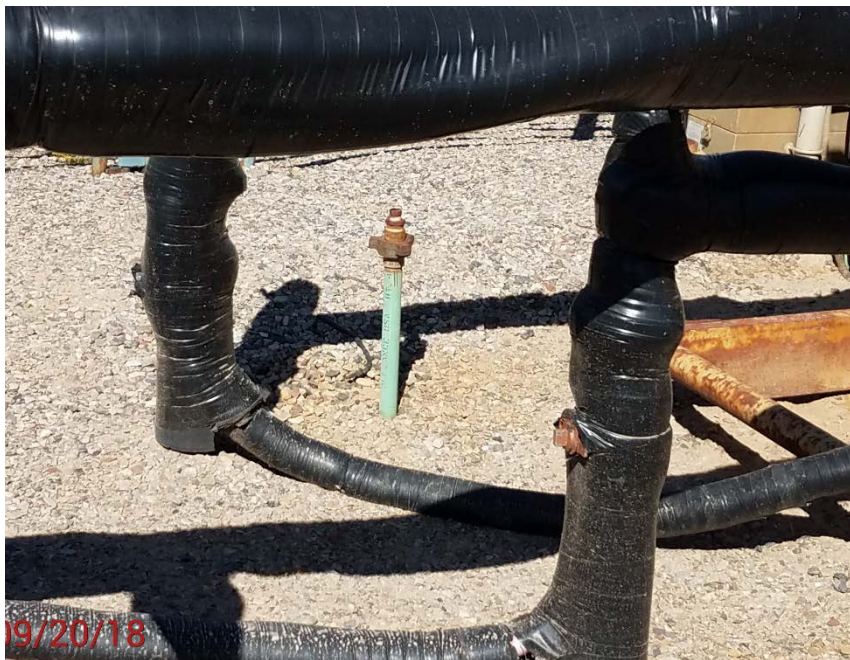
Location Photo #5, unmarked riser/flowline
