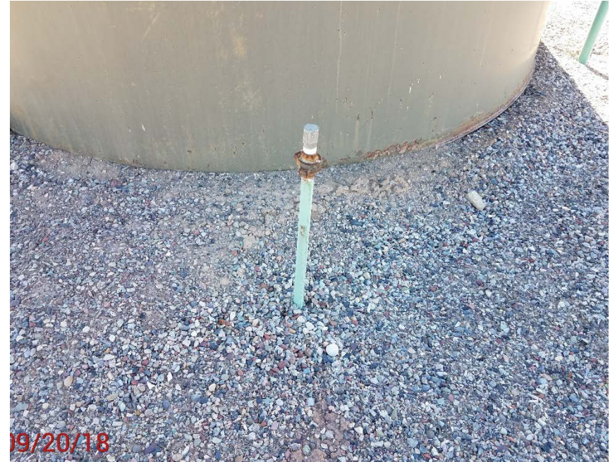
Location Photo #4, unmarked riser/flowline
