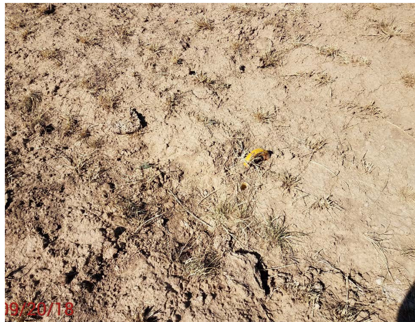
Location Photo #6, unmarked deadman anchor.
