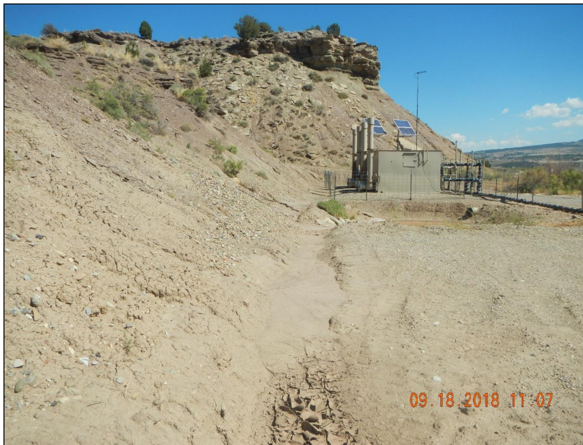
Sediment build up in ditch between tank and separators.
