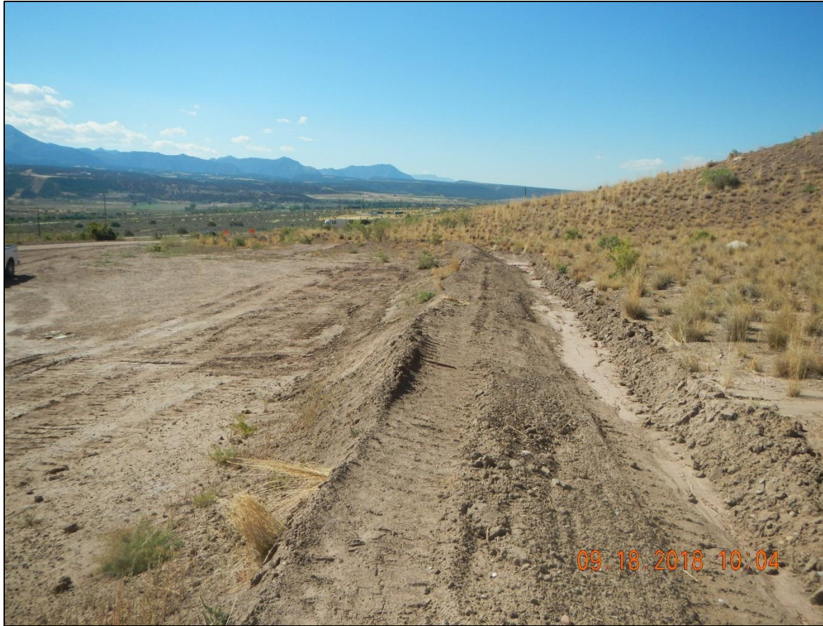
Ditch repaired on channeling and cleared of sediment.
