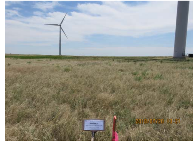
View to the south H & M Petroleum Corporation-State BDB #1, Logan County, Colorado
