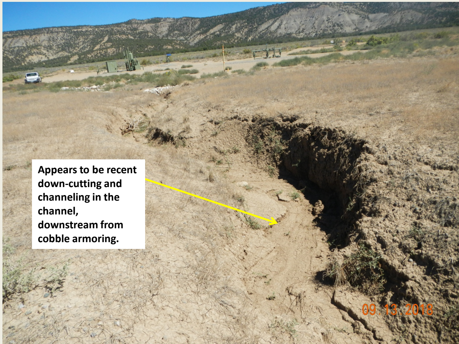
Photo 5. View of gully with cobble armoring for a portion leading from the well pad and then no armoring. It appears that stormwater flows are continuing to erode the channel. This needs to be monitored and additional stormwater controls installed if erosion worsens.
