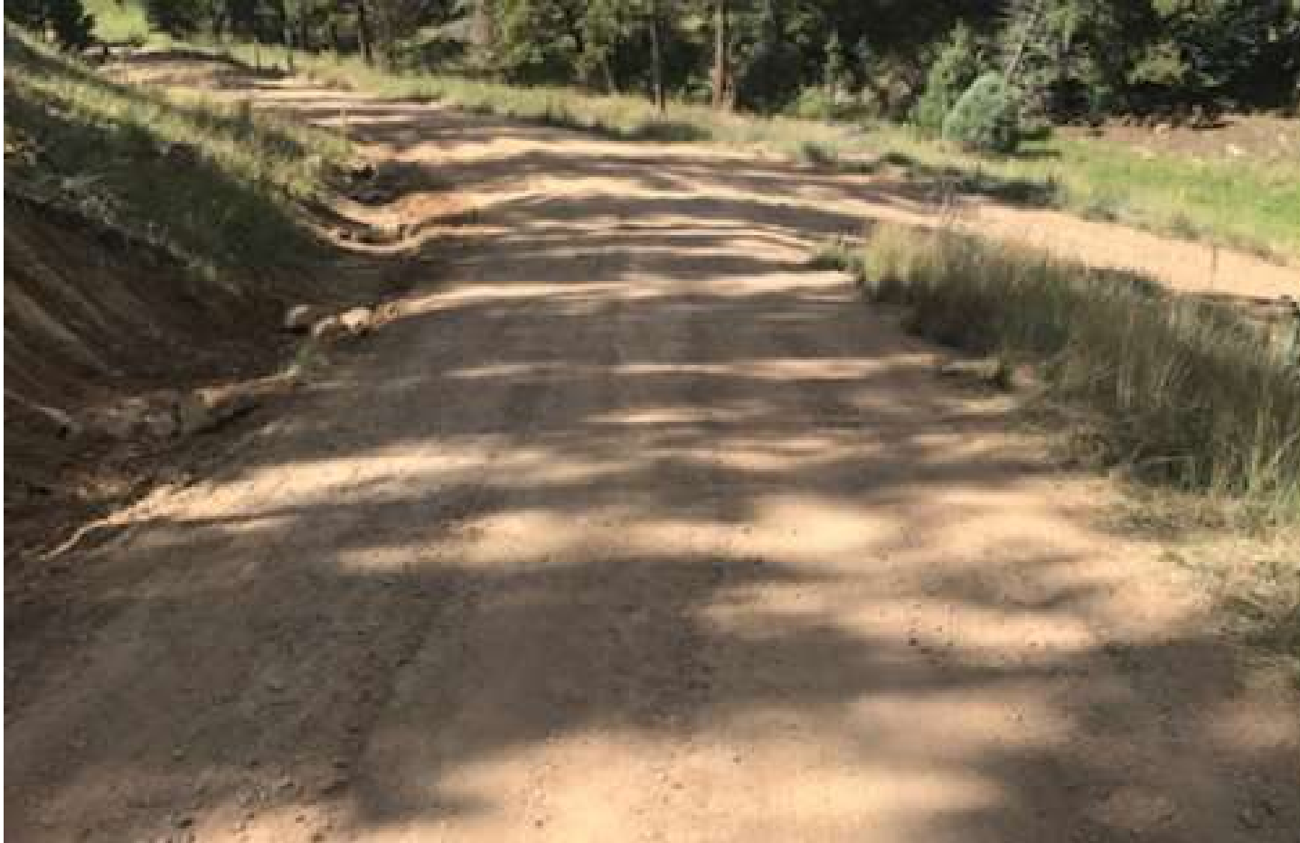
PHOTO 2: THE ACCESS ROAD TO THE WELL PAD WAS CROWNED TO ESTABLISH SHEET FLOW WHICH ELIMINATED THE SURFACE EROSION.
