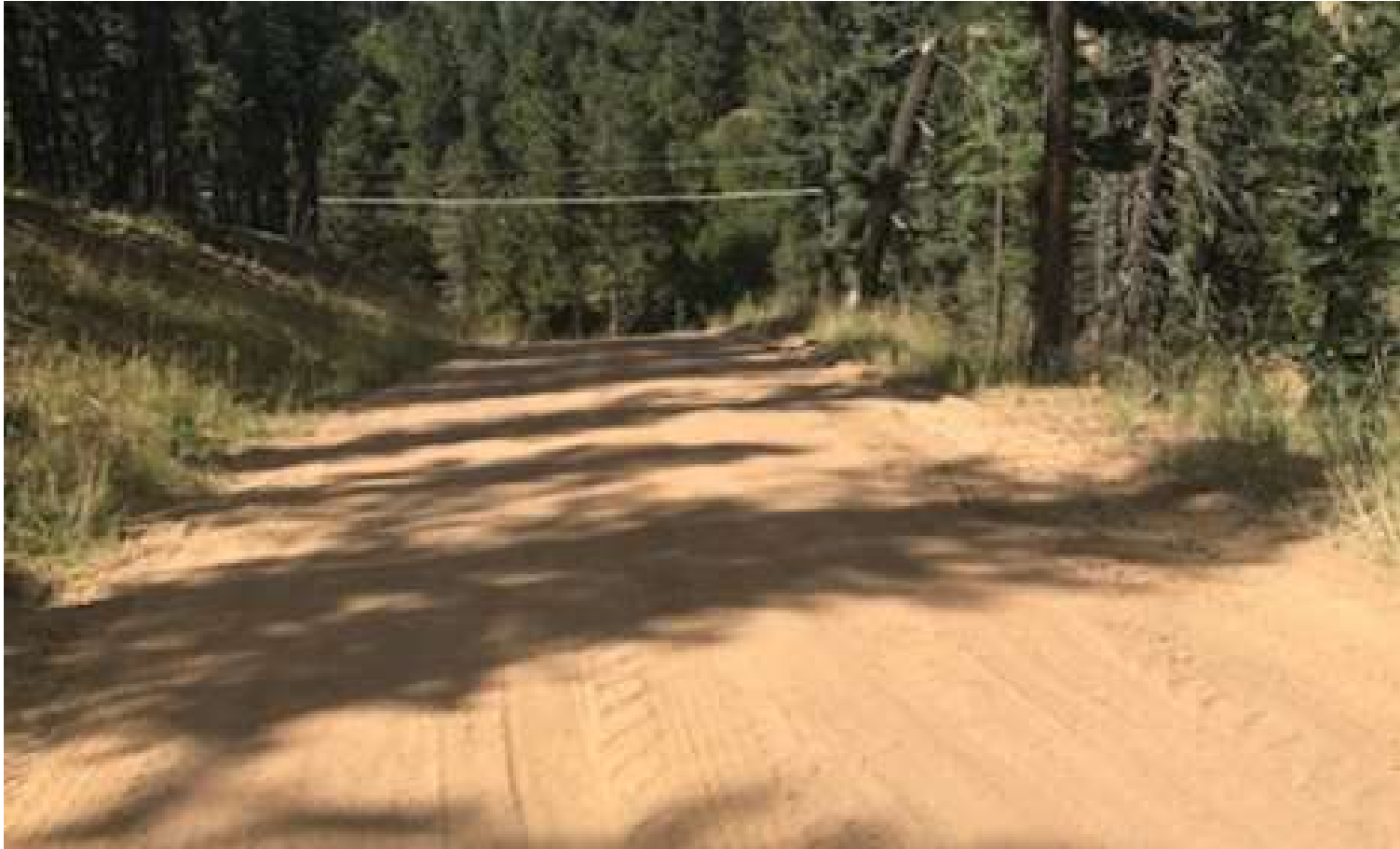
PHOTO 1: THE ACCESS ROAD TO THE WELL PAD WAS CROWNED TO ESTABLISH SHEET FLOW WHICH ELIMINATED THE TIRE RUTTING.
