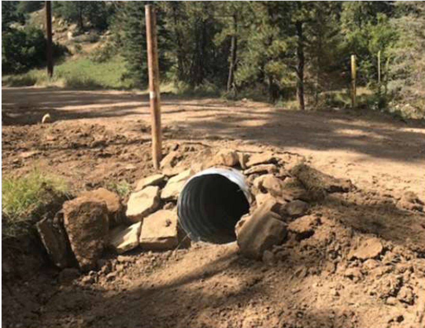
PHOTO 4: THE DAMAGED CULVERT ON THE MAIN LEASE ROAD WAS REMOVED AND A NEW GALVANIZED CULVERT WAS INSTALLED.
