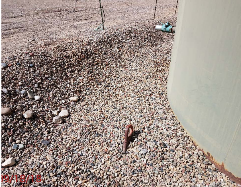
Location Photo #3, unmarked deadman near tanks.
