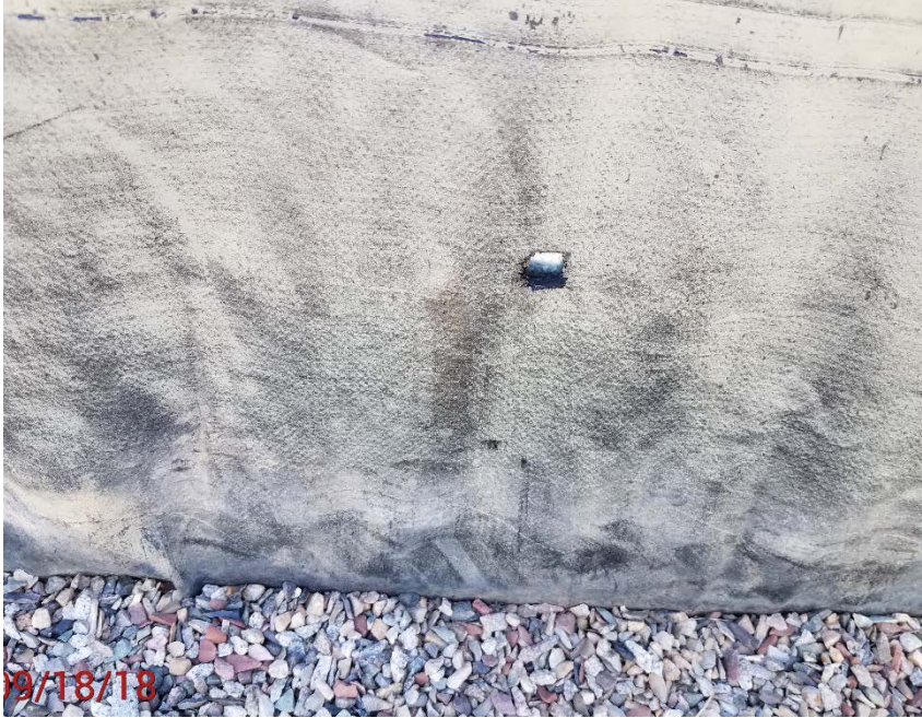
Location Photo #5, hole in battery containment liner.
