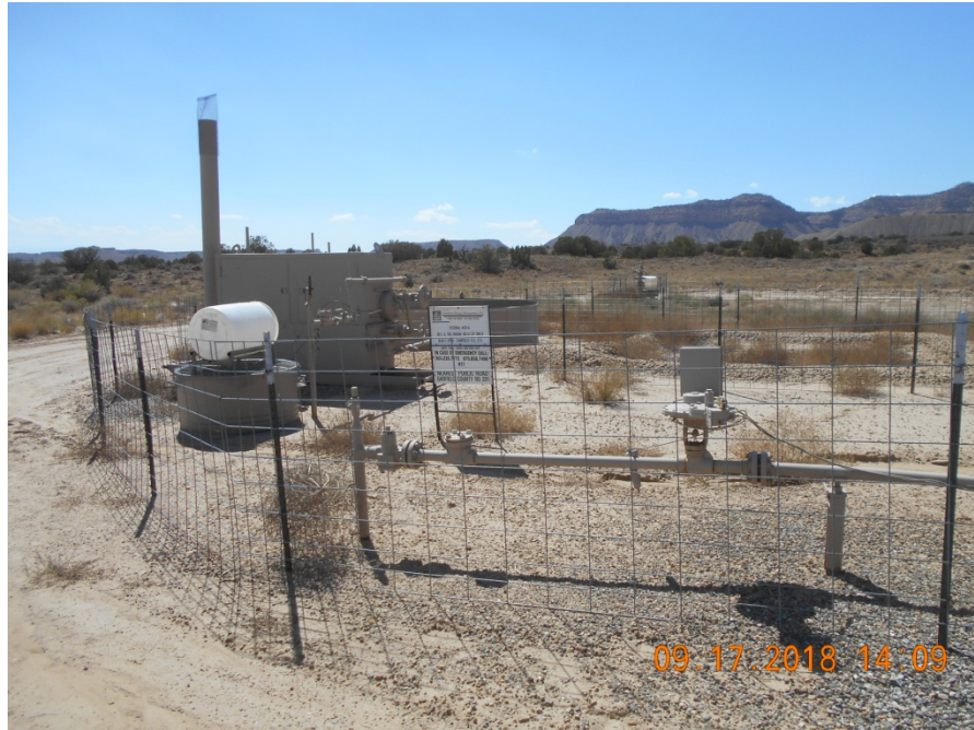
Separator, tank battery inside fencing with sign
