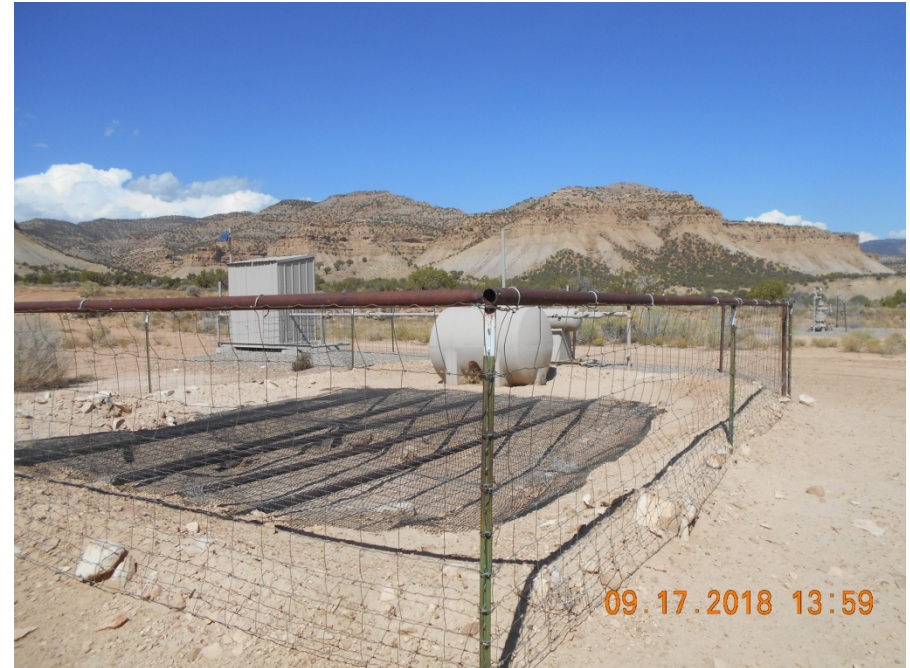
Blowdown pit and tank with fencing and mesh
