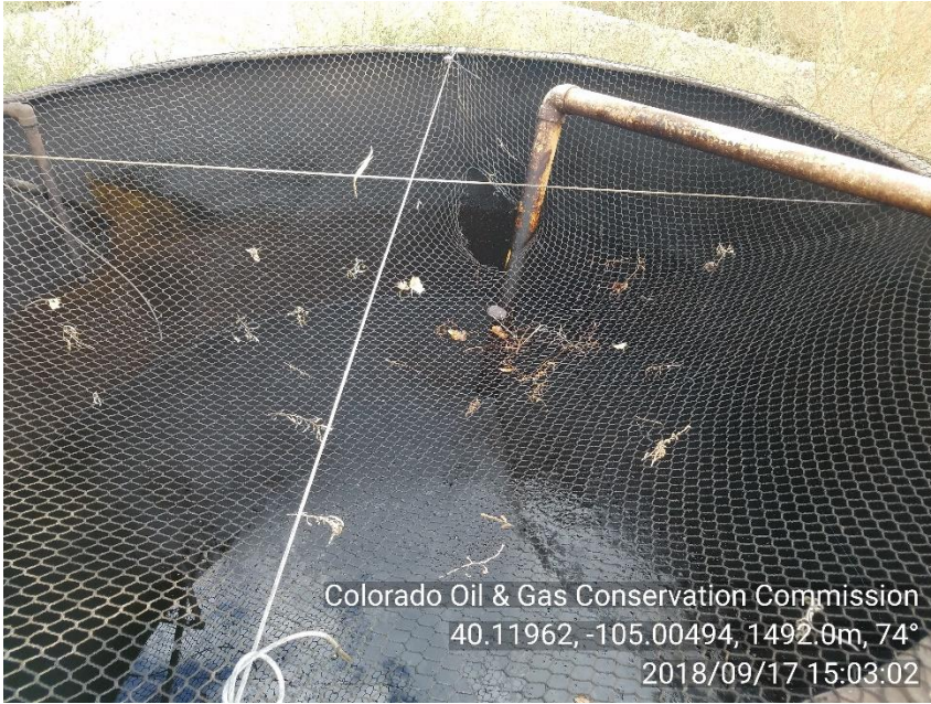
PHOTO #5: HOLE IN OPEN TOP PRODUCED WATER TANK WILDLIFE PROTECTION SCREEN
