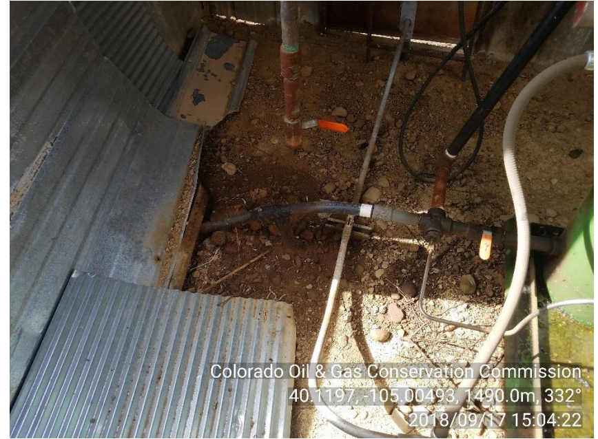
PHOTO #6: STAINED SOIL INSIDE COMPRESSOR HOUSE
