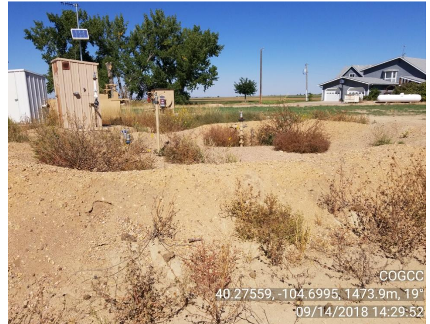
Photo 2. Locked out/tagged out flowline risers
