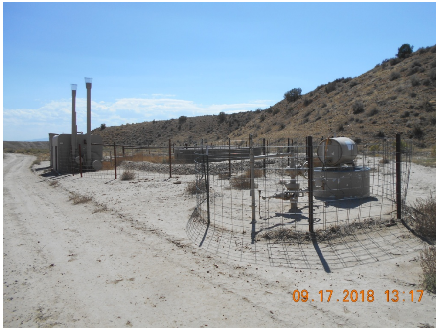
Wellhead and overview of location looking SE.
