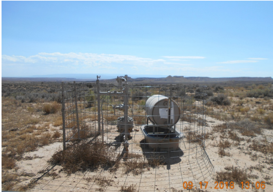
Wellhead with fencing
