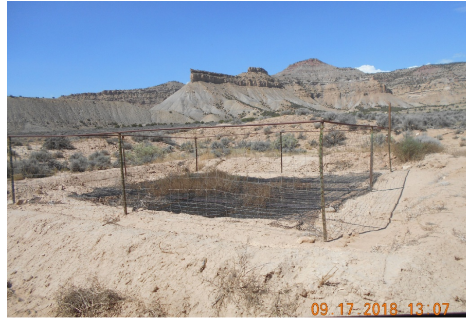
W. Side blowdown pit
