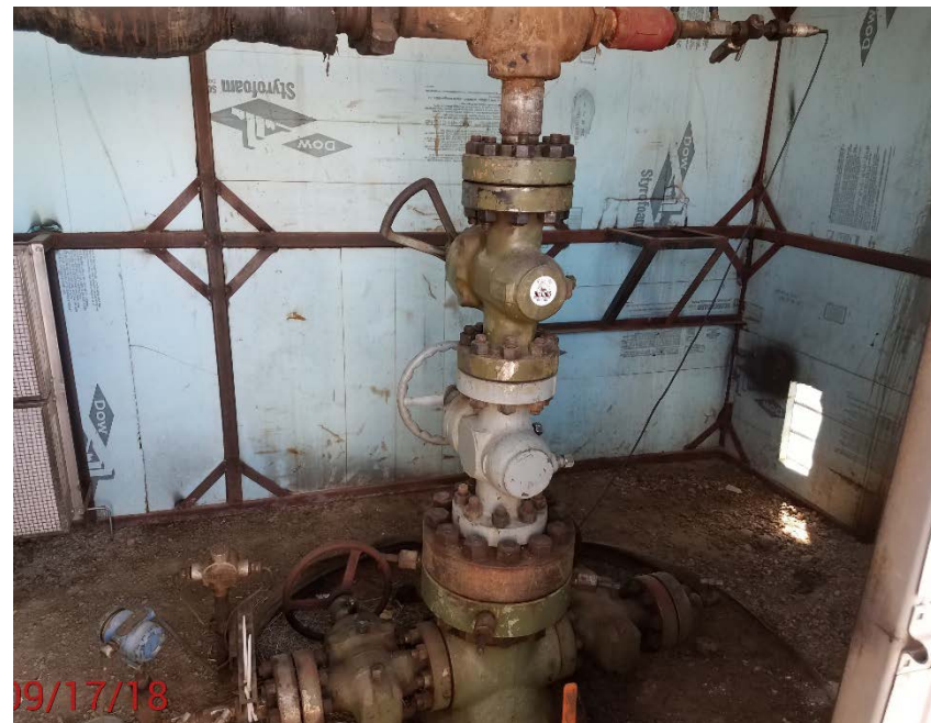
Location Photo #2, injection wellhead
