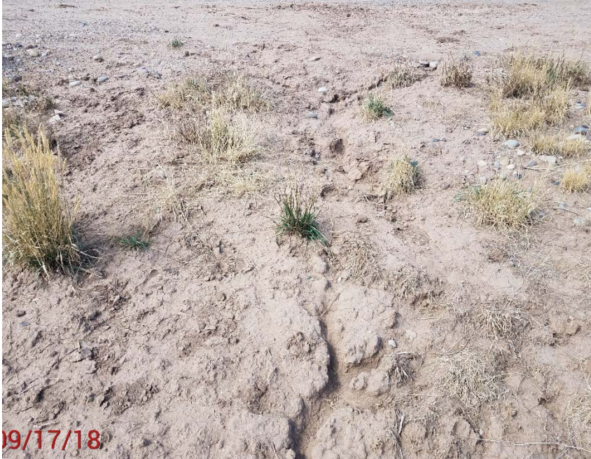
Location Photo #9, Sediment being moved off location
