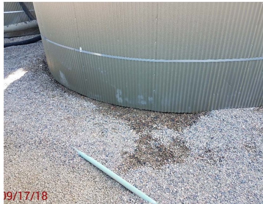
Location Photo #4, stained rock in battery containment.
