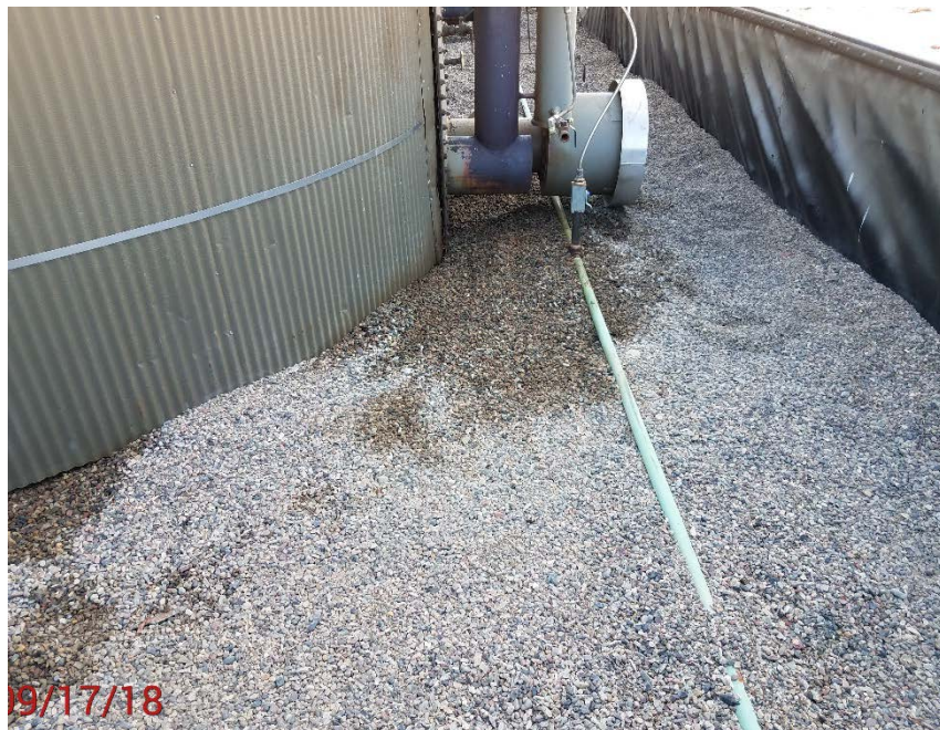
Location Photo #3, stained rock in battery containment.
