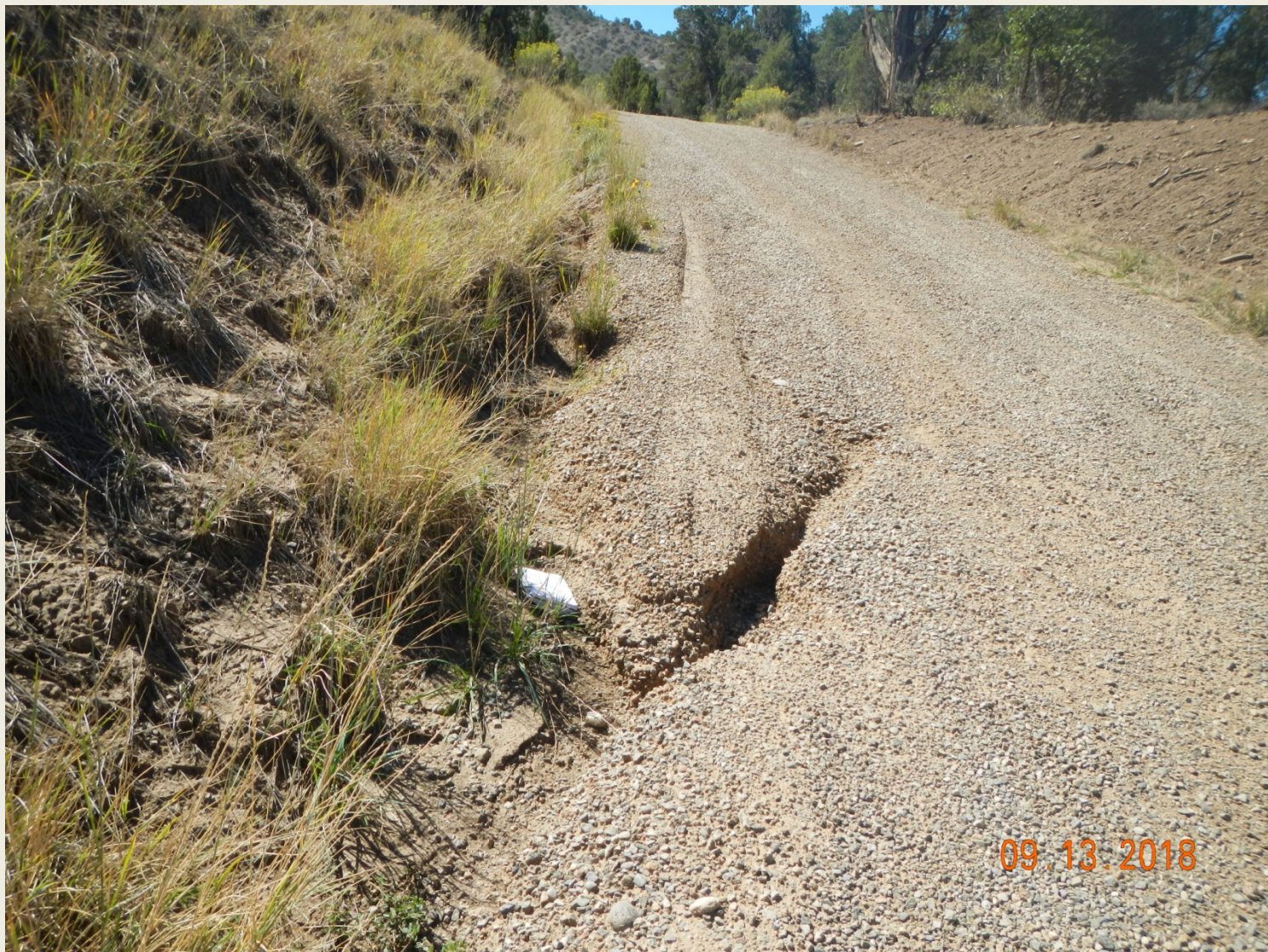
Photo 6. View of area along the access, near the well pad entrance, where stormwater flows converge and form an erosional channel that carries sediment down stream toward the well pad.
