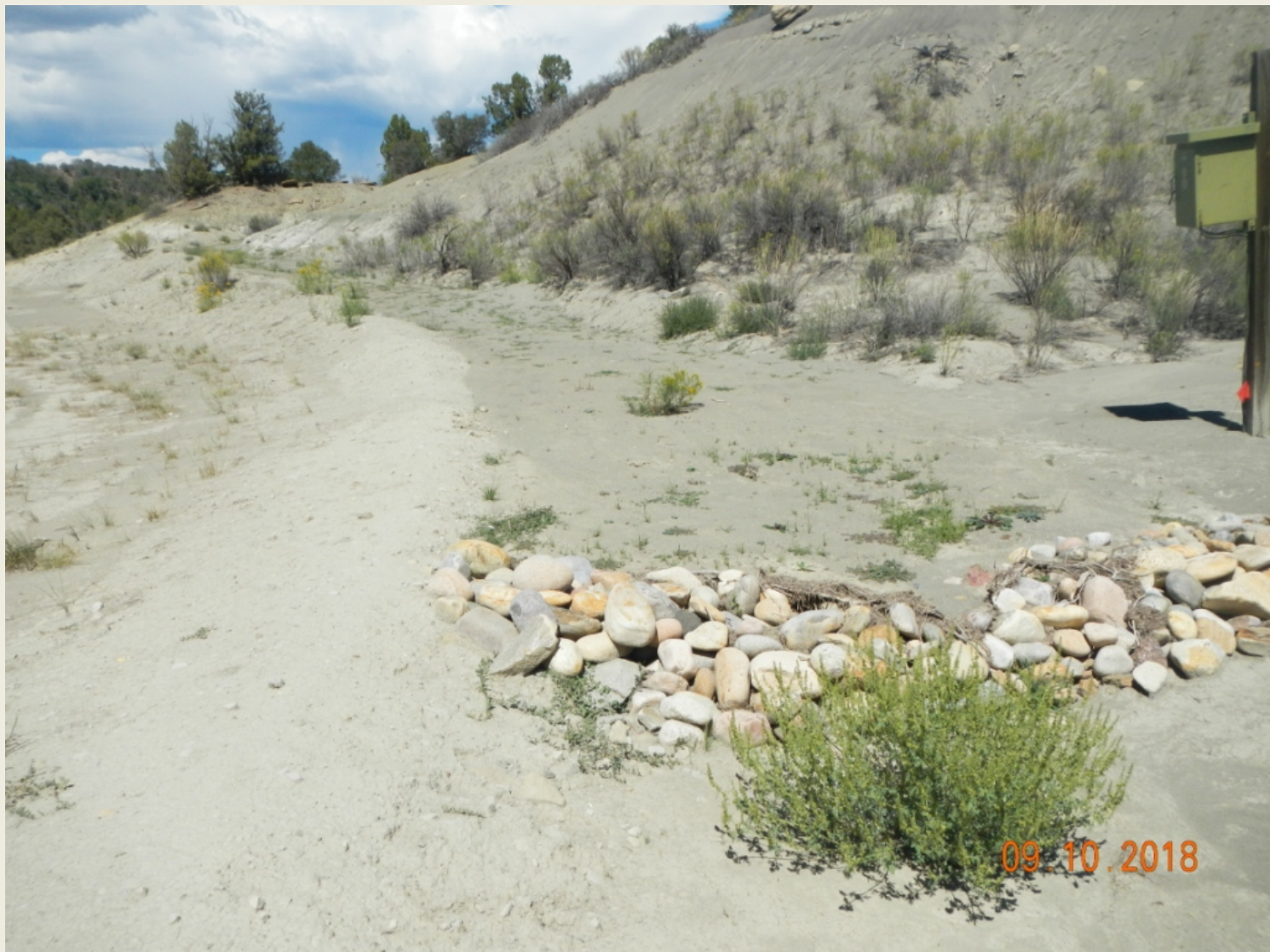
Photo 2. View of the northern project area. Cobble sediment trap is recently installed and appears to be functioning, but is full of sediment and needs maintenance. Revegetation of northern berms and cleaning sediment from diversion will help control erosion.
