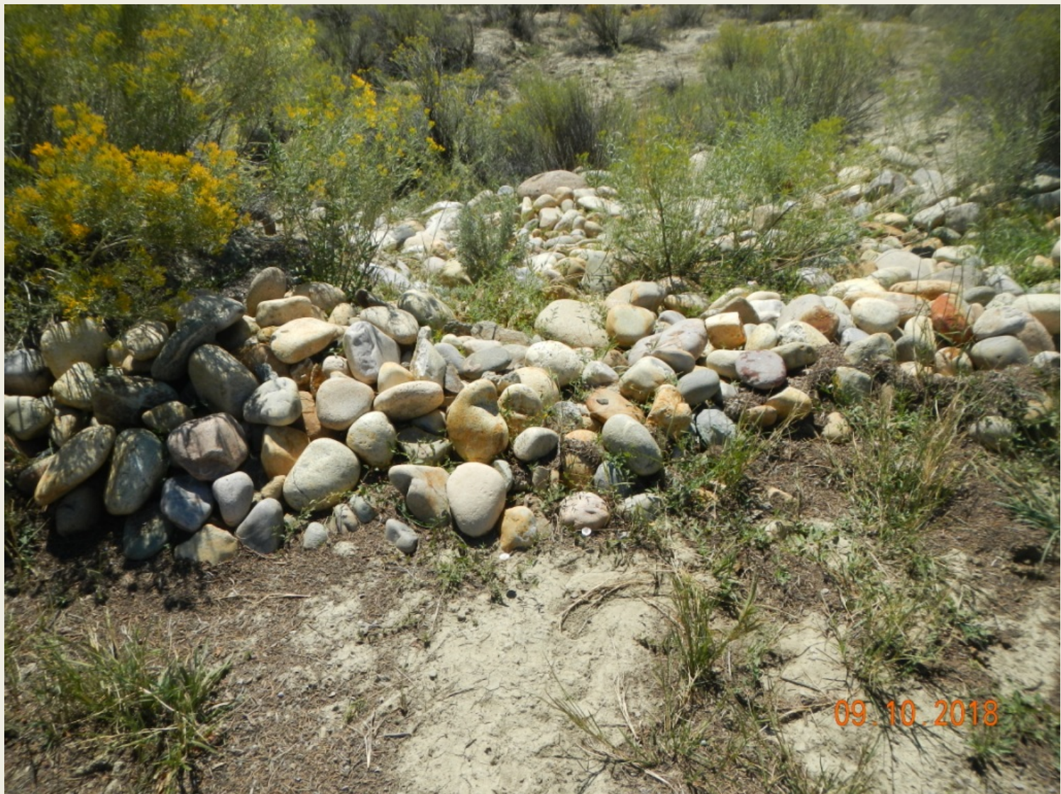
Photo 4. View of cobble run-down in the southern project area in good working condition.
