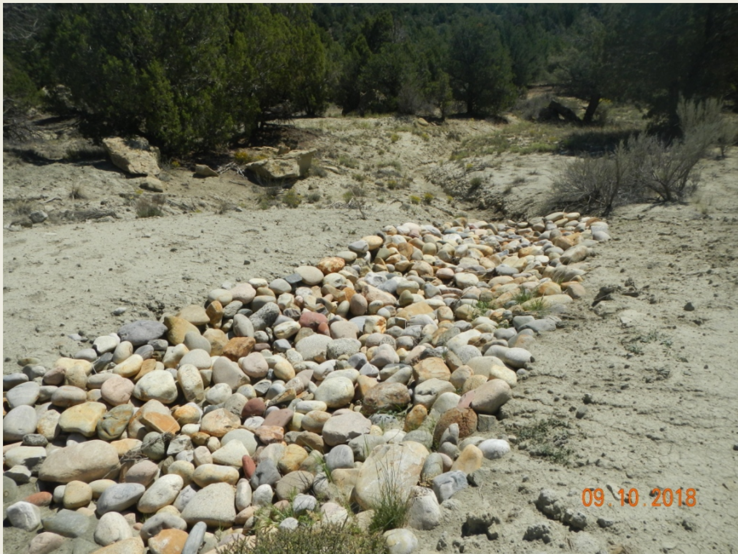
Photo 3. View of cobble run-down in the northeastern project area in good condition.
