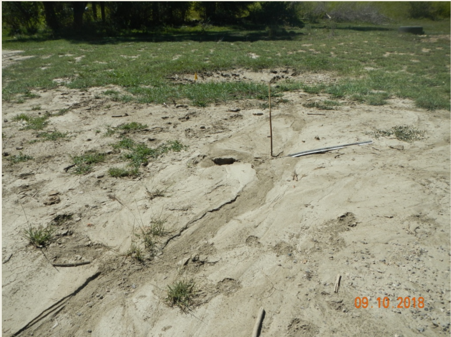
Photo 3. View of sediment deposition within the southwestern project area, downstream from photos 1 and 2. Sediment appears to be impeding desirable vegetation. Wire documented in earlier inspection is not addressed.
