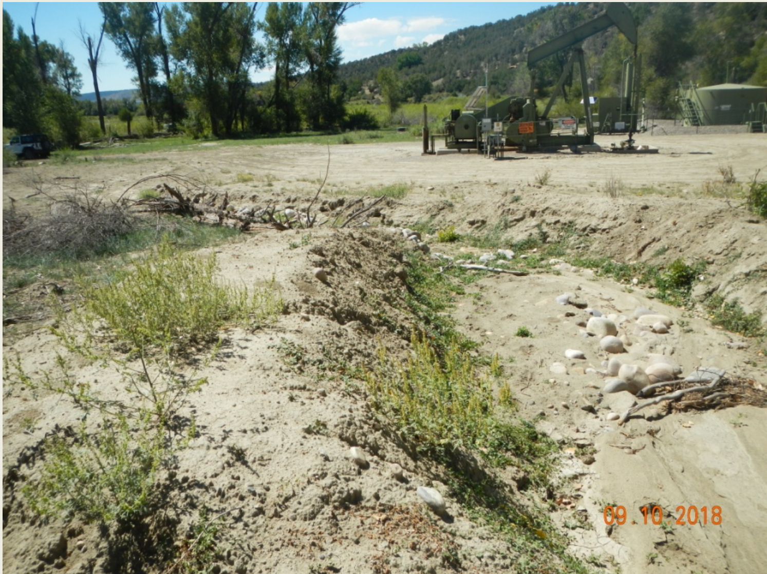
Photo 1. View of stormwater diversion with outlet on the well pad. It appears cobble was placed in the channel. Cobble is already inundated with sediment. Evidence of recent sediment deposition and stormwater flows observed on the well pad. Corrective action not addressed.
