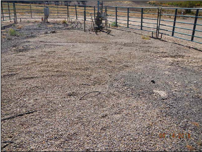
Photo 5: Stained soil has been covered or removed.
