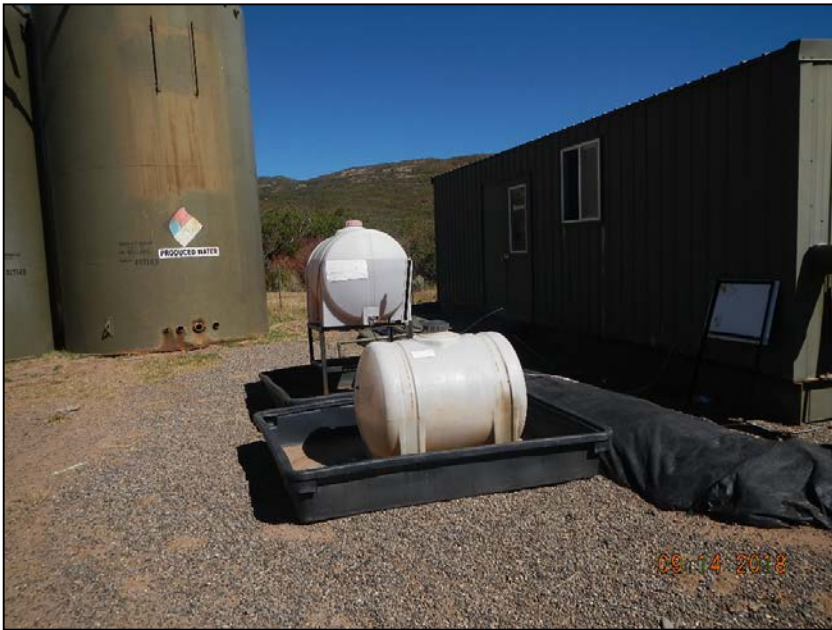
Photo 3: Chemical storage tank has been put in containment. Labels are faded and not legible.
