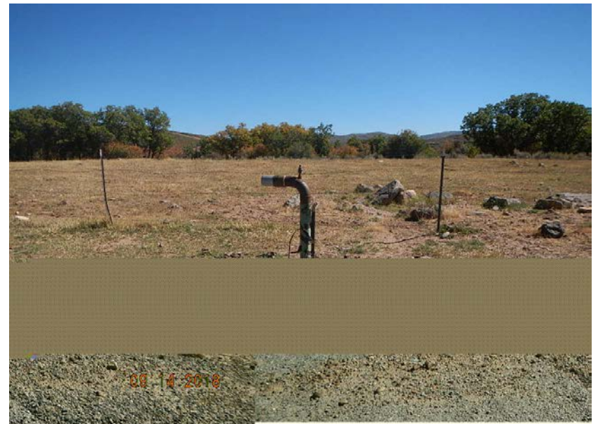
Photo 4. Risers from tank battery have not been removed.
