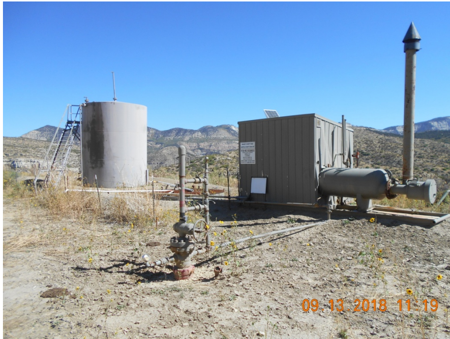
Wellhead, Separator and Tank battery
