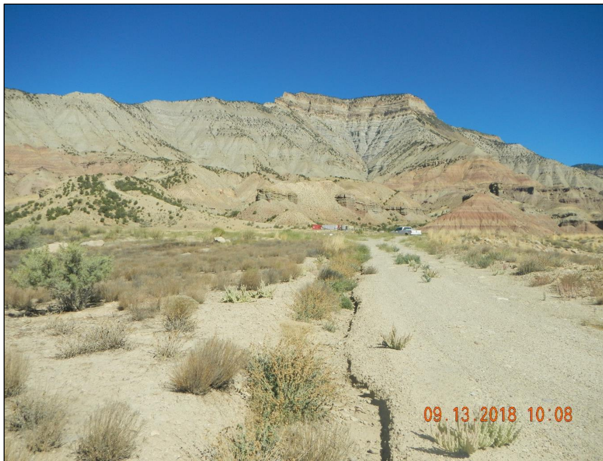
Washing and sediment movement in road ditch.
