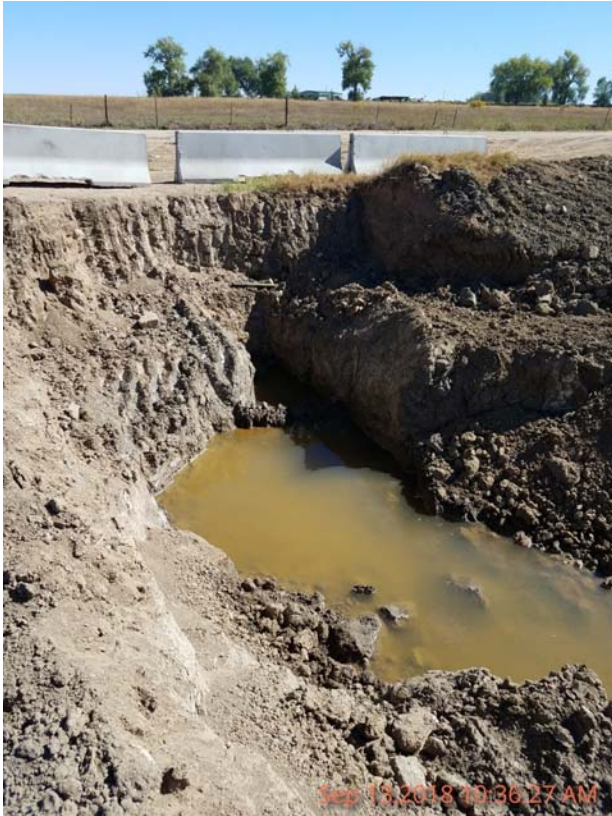
Photo 1 – Excavation exposing groundwater at Canal 2 wellhead.
