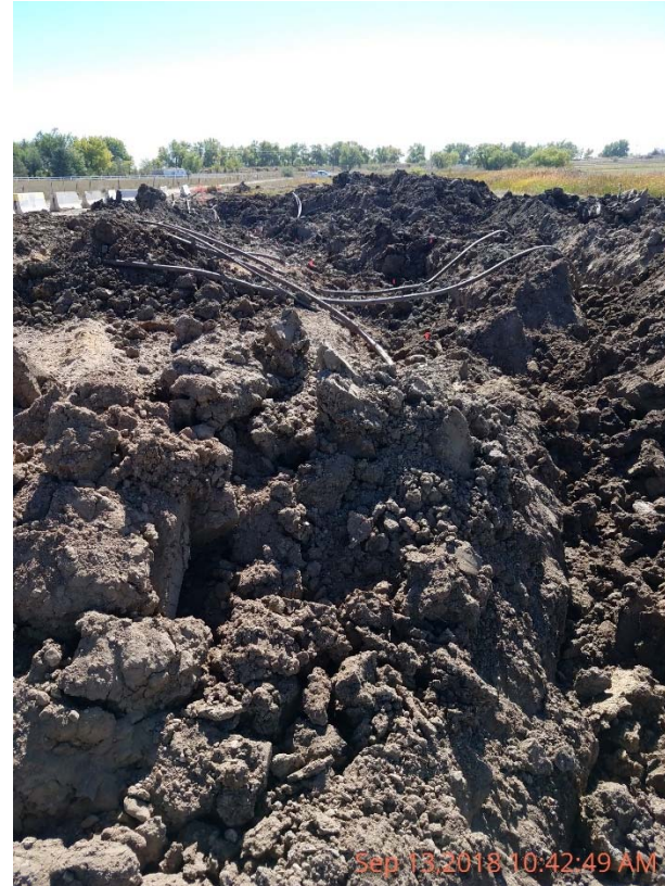
Photo 6 – Excavation of dumplines at former tank battery in progress.
