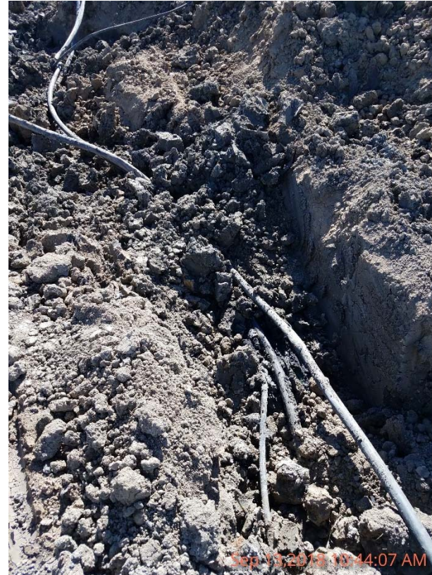
Photo 8 – Excavation exposing impacted soil at former tank battery.
