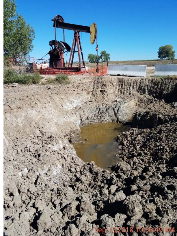
Photo 2 – Excavation exposing groundwater at Canal 2 wellhead
