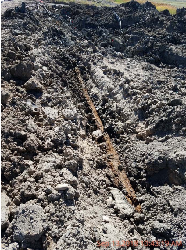
Photo 5 – Exposed dumpline trench.
