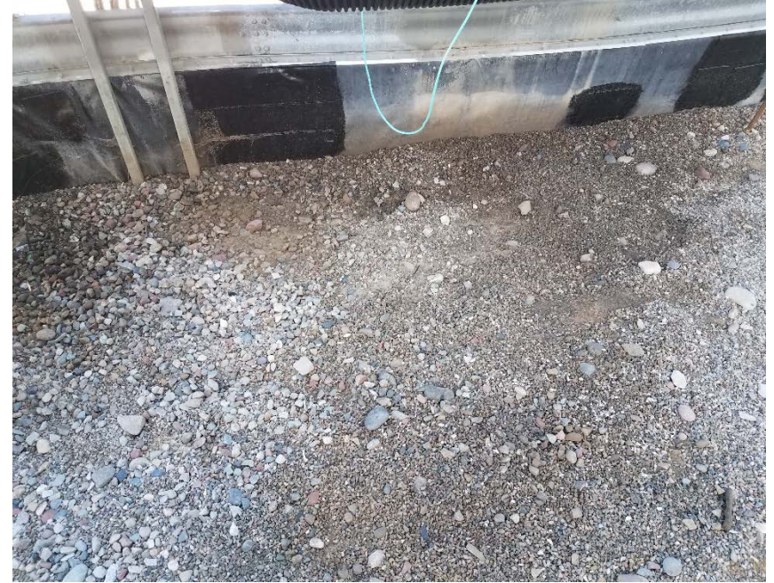
Location Photo #6, Battery containment, Patched holes.
