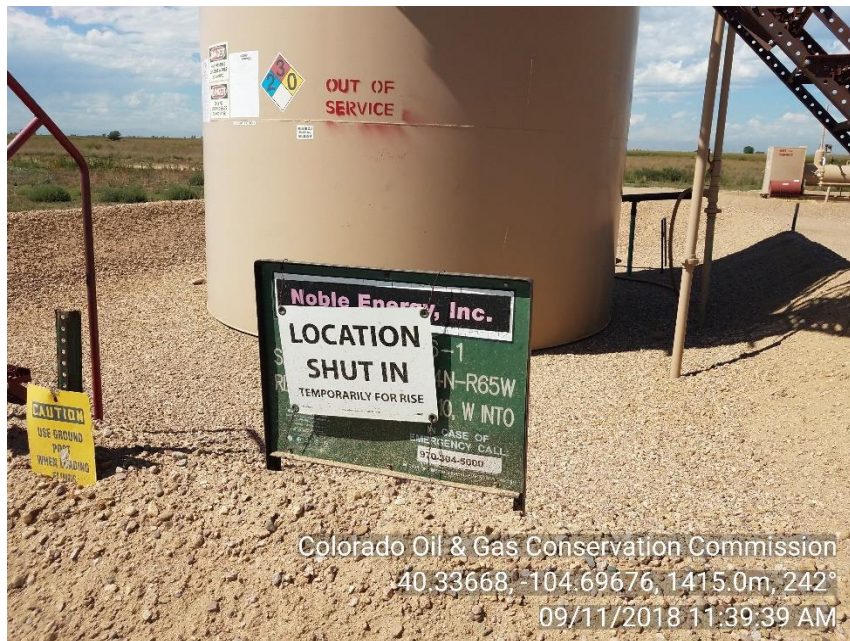
Tank battery signage
