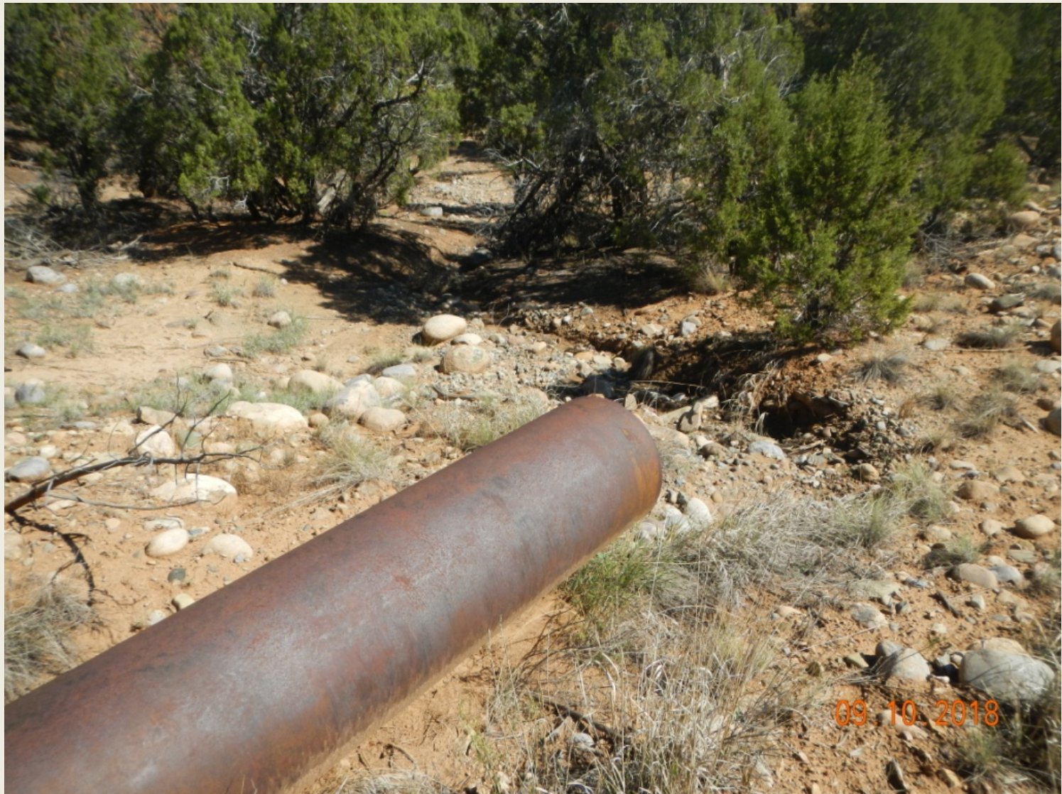
Photo 10. View of a culvert outlet along the access road where diverted flows are not properly stabilized, energy not sufficiently dispersed, and resulting in erosional channel formation downslope from the culvert.
