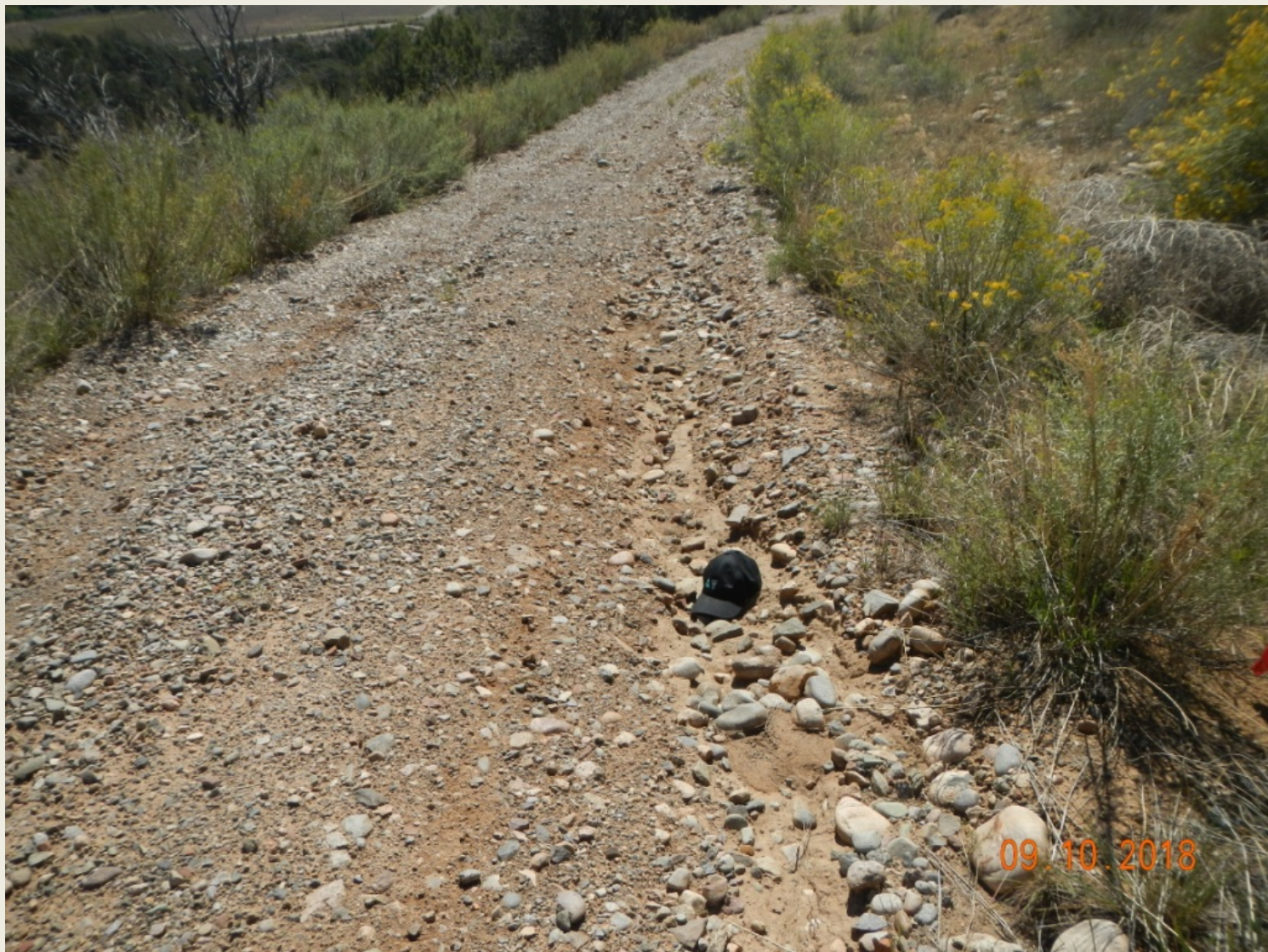
Photo 9. View of area along the access road where roadside ditch is full of sediment and stormwater flows are diverted to the road surface, causing erosion along the road.
