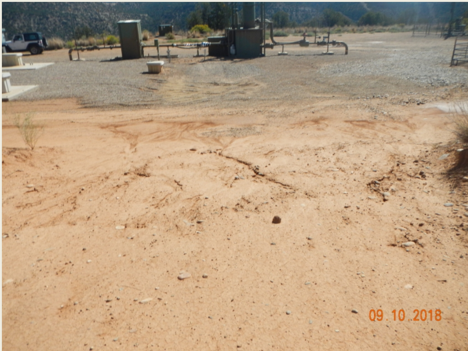
Photo 7. View of sediment deposition on the well pad from disturbed soils within the western project area.
