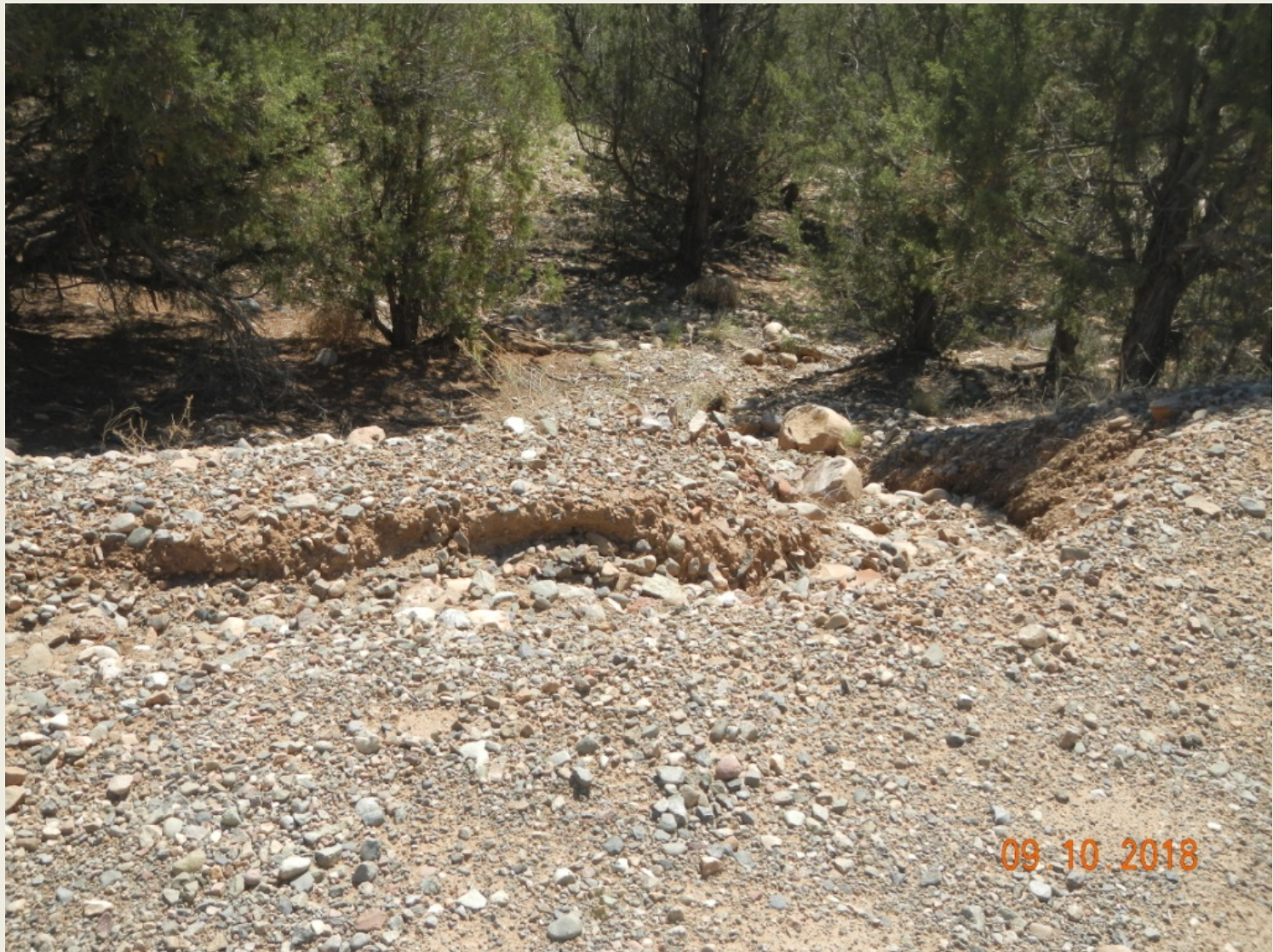
Photo 8. View of erosional channel forming on the access road where improperly diverted stormwater is eroding the road and downslope.
