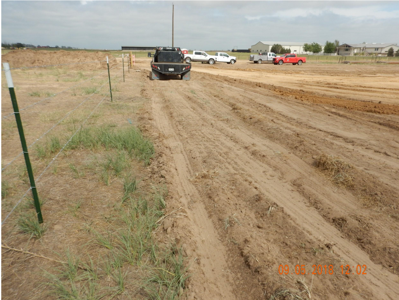
Photo 4. Photo taken from the northwestern location, facing North. Operator is driving over the top of the BMP. Operator shall keep off BMPs so they remain in proper functioning condition. Operator indicated that surface roughening BMPs are re-ripped every 2 days due to vehicle and equipment traffic.
