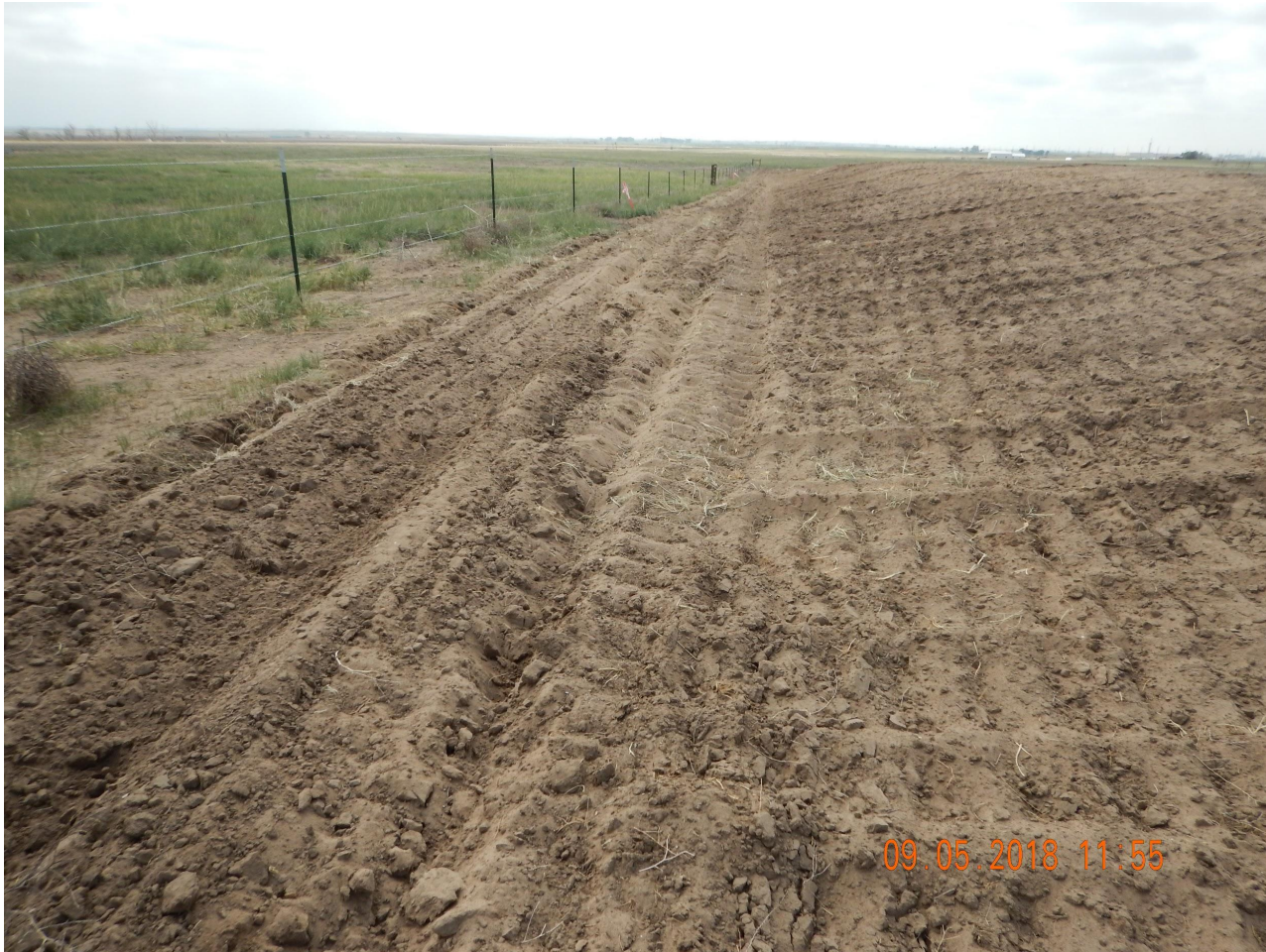
Photo 1. Photo taken from the northeastern location, facing South. Surface roughening BMP installed around portions of the perimeter location. This location is very sandy and will require more appropriate BMPs than surface roughening. Operator indicated that the entire disturbance area would be hydromulched and seeded upon completing the pad construction. Photo also illustrates the topsoil stockpile that has been temporarily stabilized with equipment tracking.
