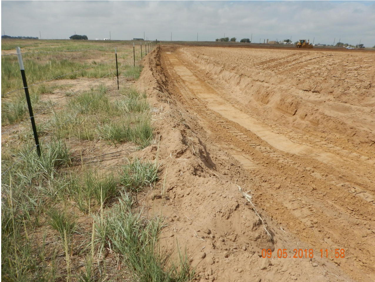
Photo 2. Photo taken from the southeastern location, facing West. Appears a retention pond has been constructed. Operator indicated pad will be sloped (0.5%) towards the south to allow for proper drainage. See comments under Photo 1.
